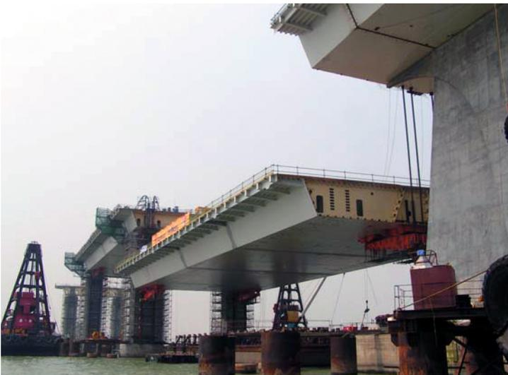
Figure 8: Lifting of Back Span
