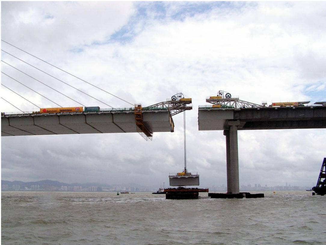
*Figure 10: Lifting of the Main Span Closure Segment*
