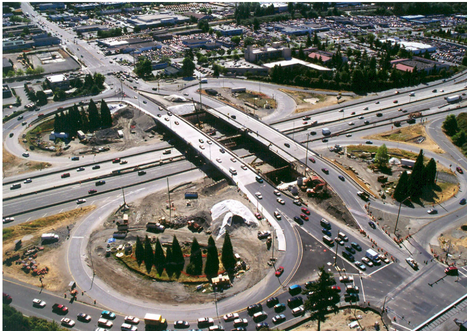
Figure 1 – The Northeast 8 th Street bridge prior to rolling the south half-bridge into its permanent position. Eastbound traffic jogs to the right to cross over I-405 on the south half-bridge. Westbound traffic travels straight across I-405 on the new north half-bridge. The permanent south abutments and center pier are in the gap between the south half and north half superstructures.
