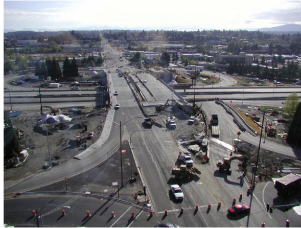
Figure 2 – The new Northeast 8 th Street bridge with the south half-bridge rolled into its permanent location. The temporary approach roadway that no longer connects to the relocated bridge is at right.
