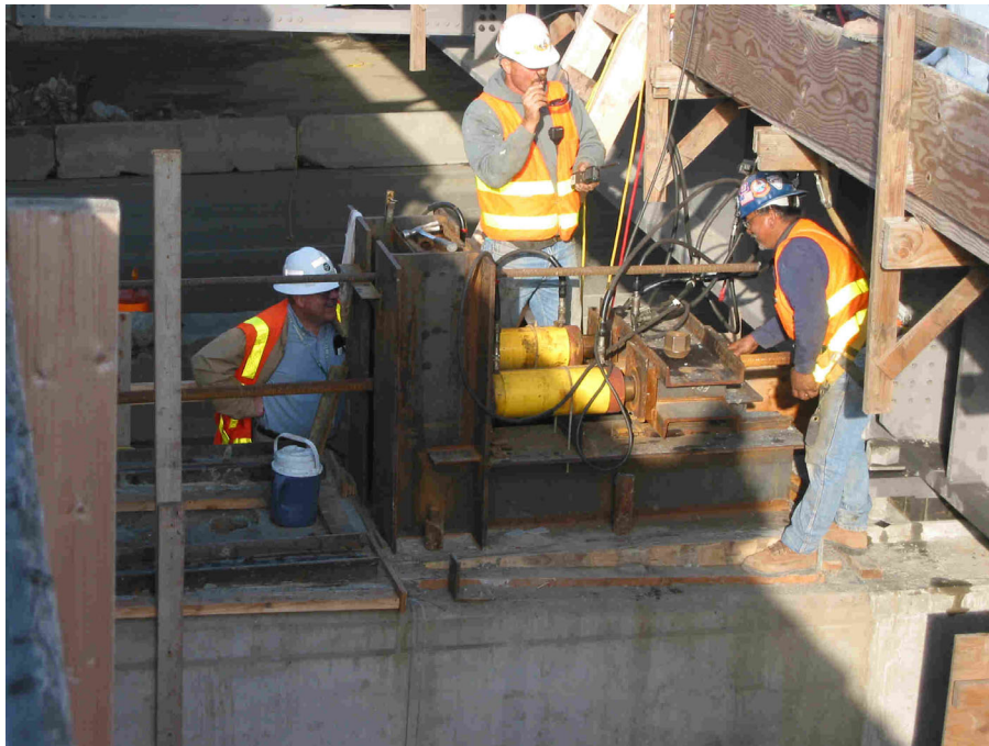
Figure 5 – Bridge rolling: The worker at far right manually tightens the nut that locks the pull rod to the jacking beam. The two jacks bear against the L-shaped, steel reaction frame, thereby pushing the jacking beam and pulling the bridge structure as the jacks extend.
