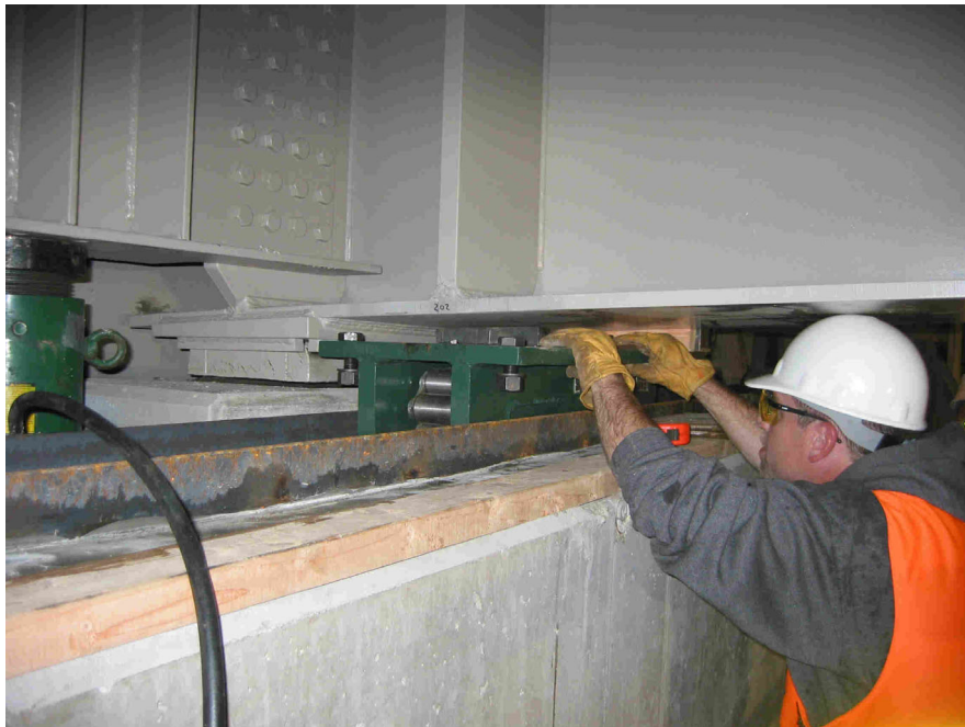
Figure 6 – With the bridge lifted by hydraulic jacks, a roller is aligned under the girder.
