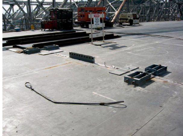
Fit-up lugs are needed to facilitate field assembly.
