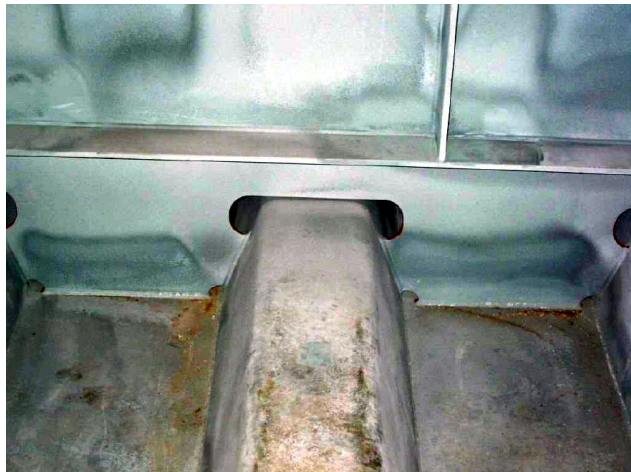
Typical closed ribbed orthotropic deck segments.
