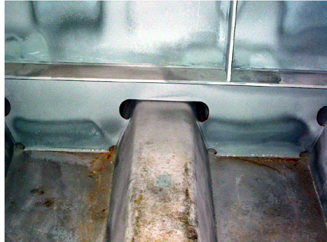
State of the art details provide good fatigue life in orthotropic steel bridges.
