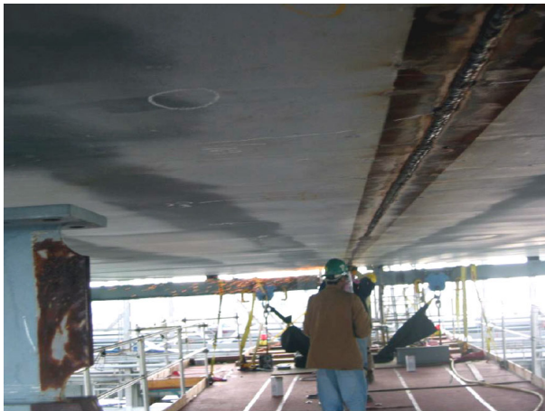
Full penetration field welds, versus partial penetration welds, facilitate non-destructive testing.
