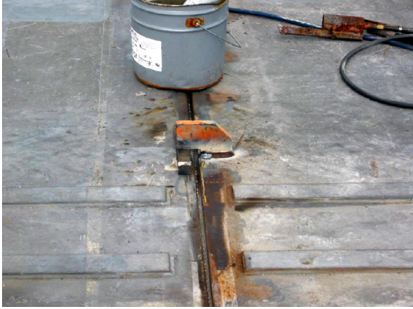
Fit-up lugs are needed to facilitate field assembly.
