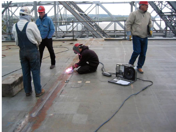
Full penetration field welds, versus partial penetration welds, facilitate non-destructive testing.
