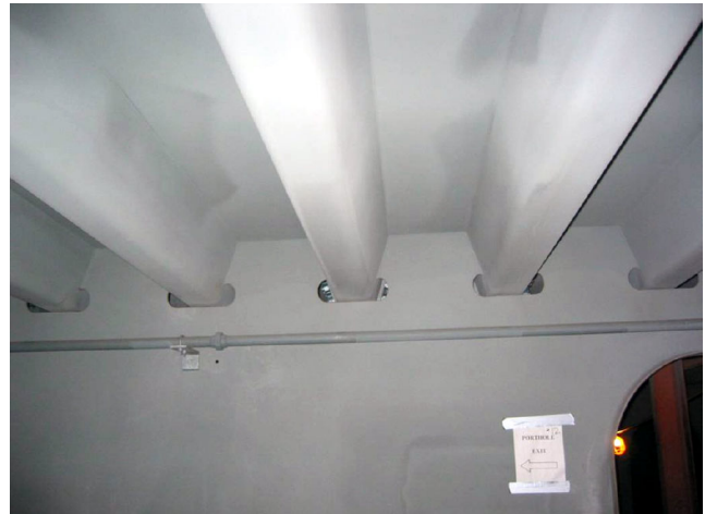
Typical closed ribbed orthotropic deck segments.
