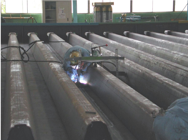
Rib to deck tack welding.
