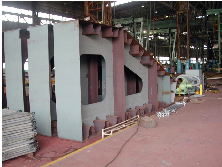
Shop assembly should be required for field units, especially for suspension bridges.
