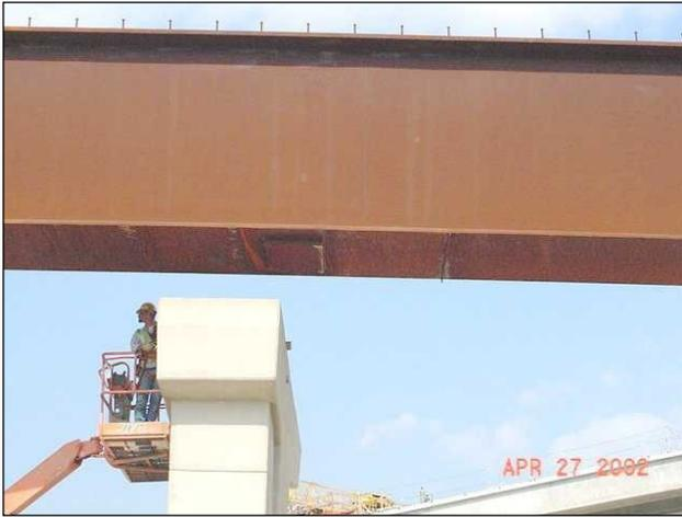
**Figure 6. Steel Tub Girder Being Lowered in Place at an Interior Bent, IH 35 / US 71 / US 290 Interchange in South Austin, Texas (note the beveled sole plate); During Construction (April 27, 2002).**
