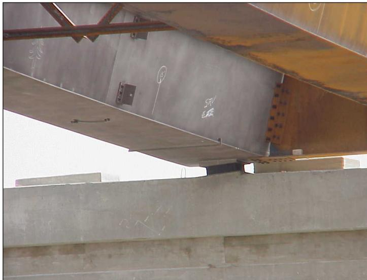
**Figure 2. US 290 / IH 35 Interchange, Direct Connector "Z", Steel Tub Girder Unit #1 End Bearing, Under Construction (03-07-2000).**
