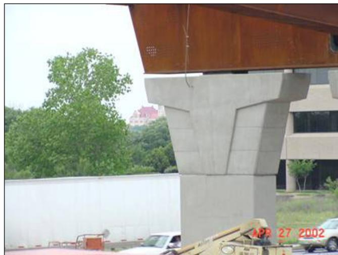
**Figure 8 Elastomeric Bearing Supporting a Steel Straddle Bent Supporting Four Steel Tub Girders, IH 35 / US 71 / US 290 Interchange in South Austin, Texas; During Construction (April 27, 2002).**
