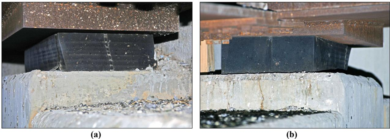
**Figure 10. East End of South IH 35 to East US 71 / US 290 Direct Connect Steel Tub Girder Unit, Showing (a) South End of North Bearing and (b) North End of South Bearing; Ready for Service (09-12-2005).**
