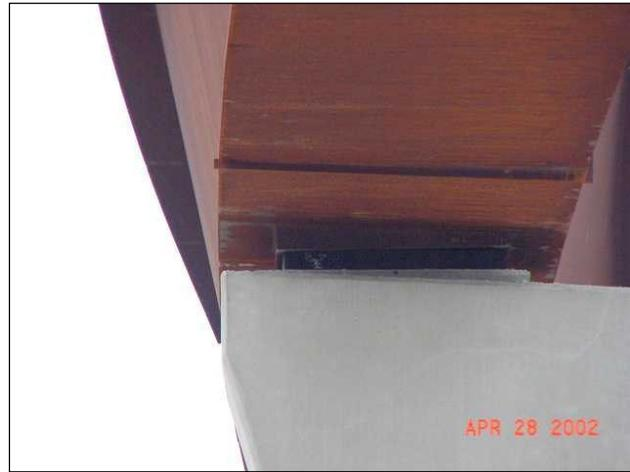
**Figure 7. Steel Tub Girder and Bearing in Place at an Interior Bent, IH 35 / US71 / US290 Interchange in South Austin, Texas (note the beveled sole plate); During Construction (April 28, 2002).**
