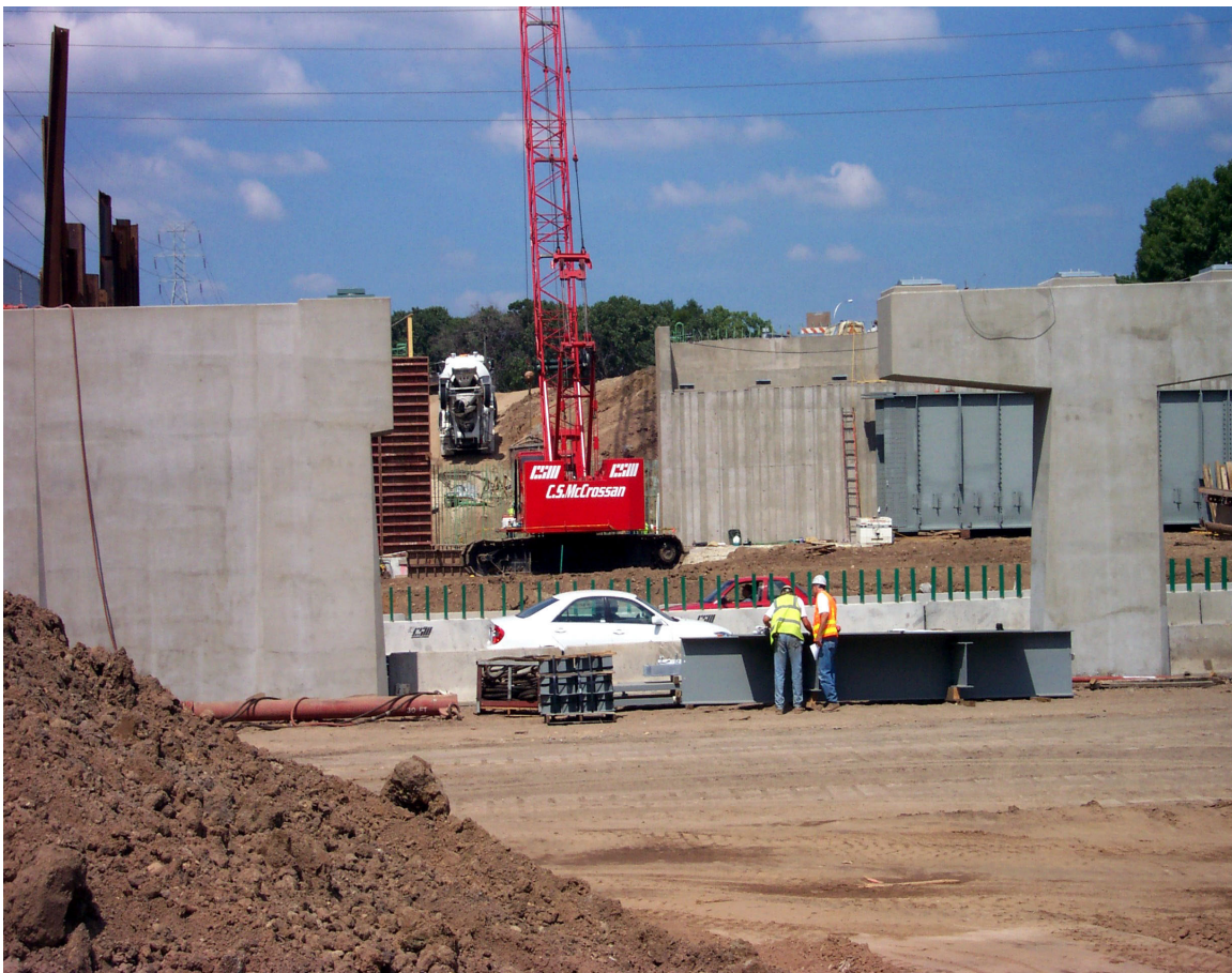
Figure 1: Railroad Bridge Girders on Site of Vehicular Bridge
