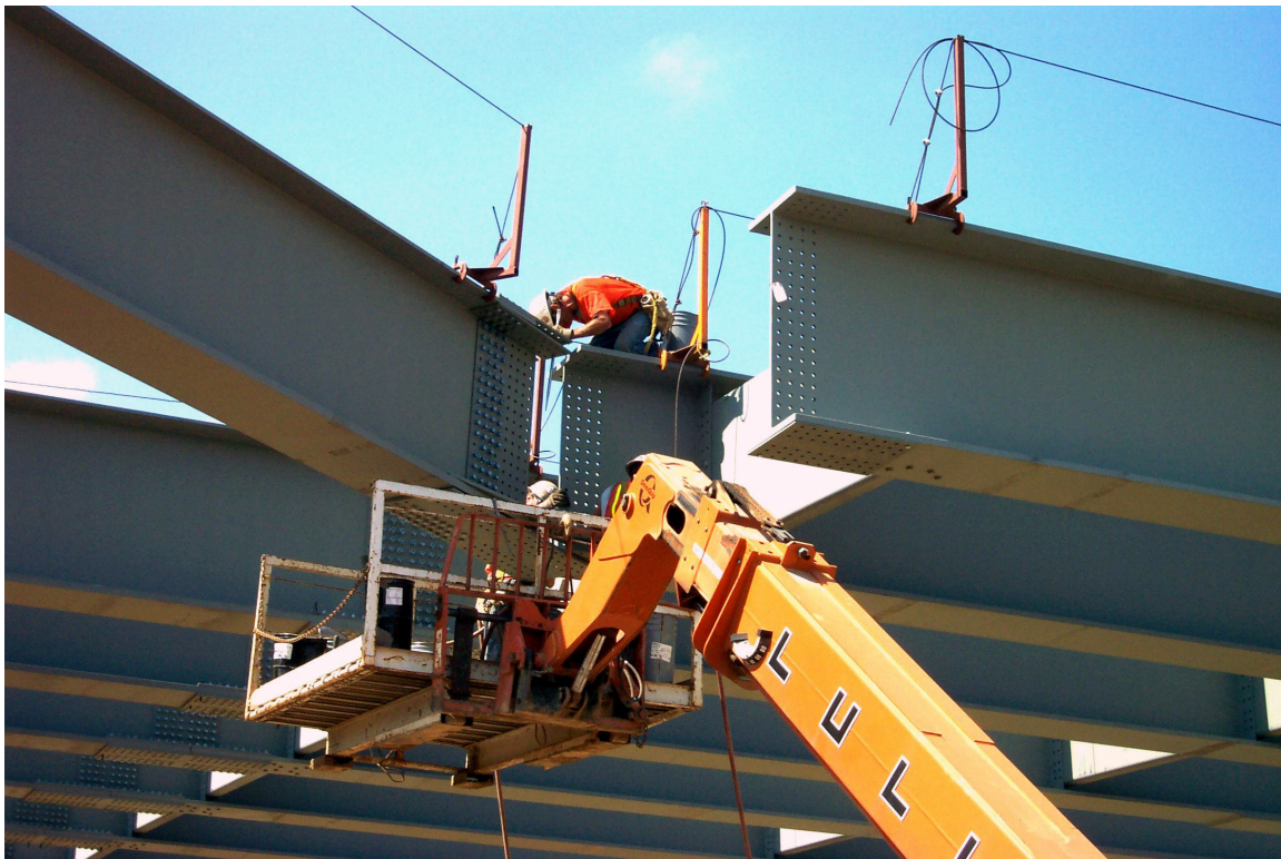
Figure 4: Assembling a Field Splice
