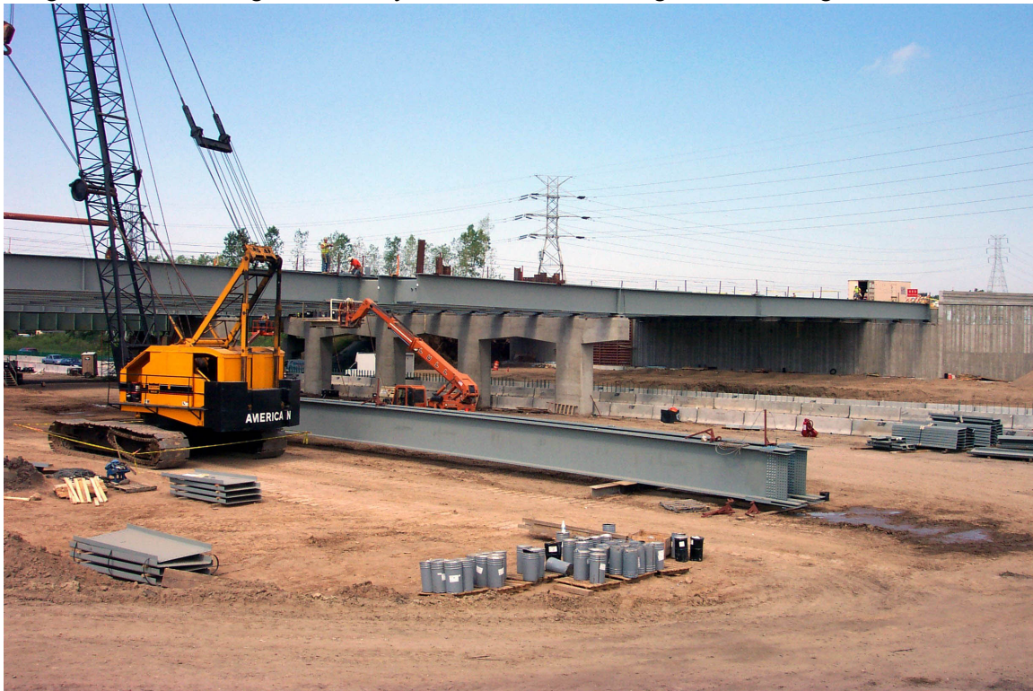
Figure 3: Girder Assembly and Erection of Vehicular Bridge
