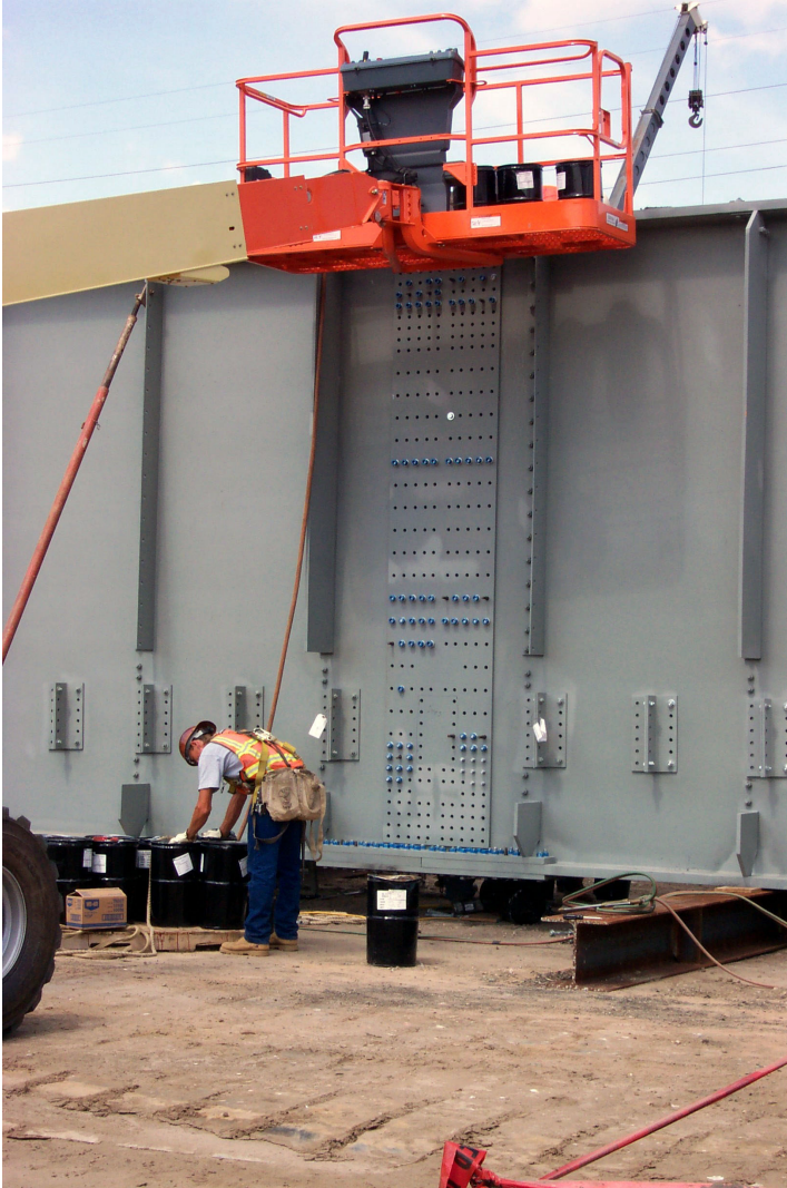
Figure 2: Assembly of Railroad Through Girders
