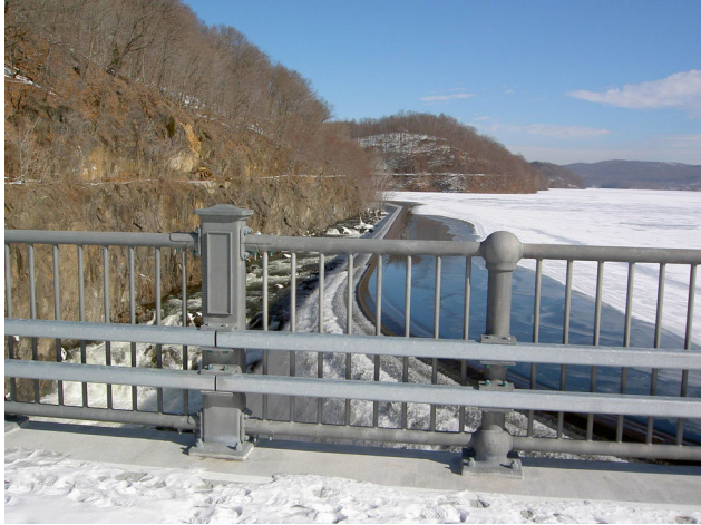
Figure 12: Main and Secondary Posts of the New Bridge Railing
