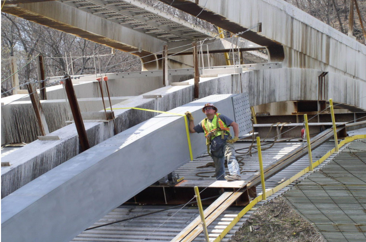
Figure 13: Erection of New Bridge Using Existing Bridge as Shoring
