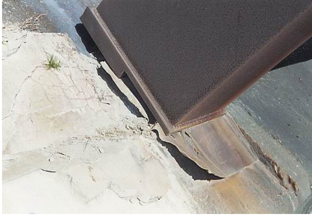
Figure 5: Arch Base displacements of the 1975 bridge were up to 14 inches
