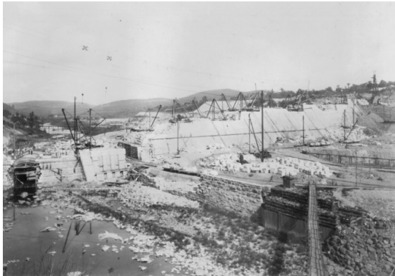
Figure 1: Historic New Croton Dam under Construction Circa, 1900
