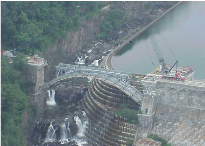
Figure 13: Erection of New Bridge Using Existing Bridge as Shoring
