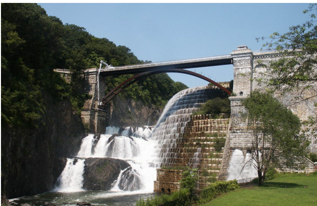
Figure 4: Open Spandrel Arch Bridge completed in 1975
