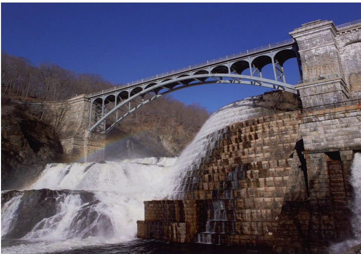
Figure 15: Completed Context Sensitive Replacement Bridge
