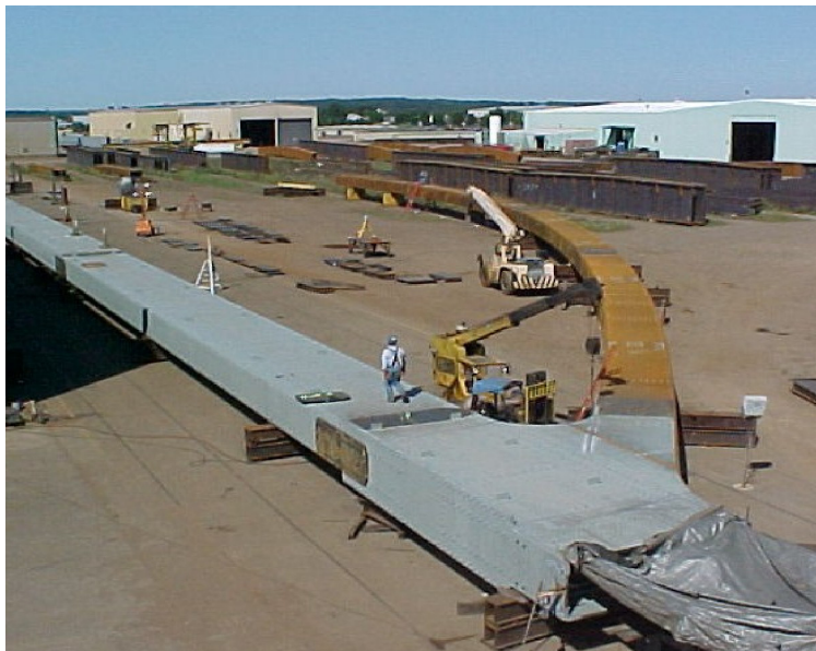
Figure 11 Arch Check Assembly
