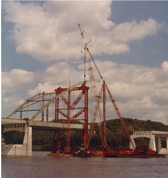
Figure 12 Arch Erection with Falsework
