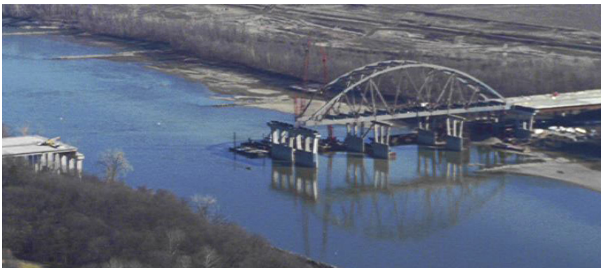
Figure 15 Route 364 Arch - Initial Erection on Approach Piers
