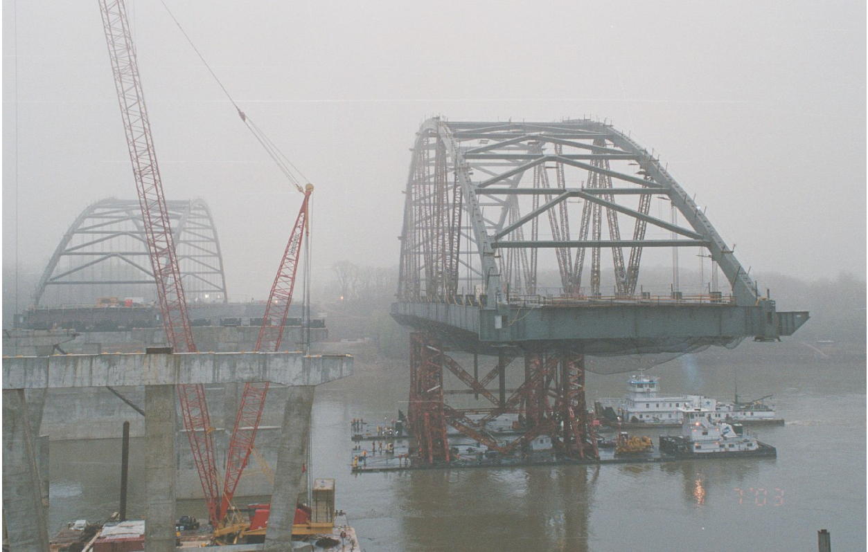
Figure 16 Route 364 Arch - Float In Operation
