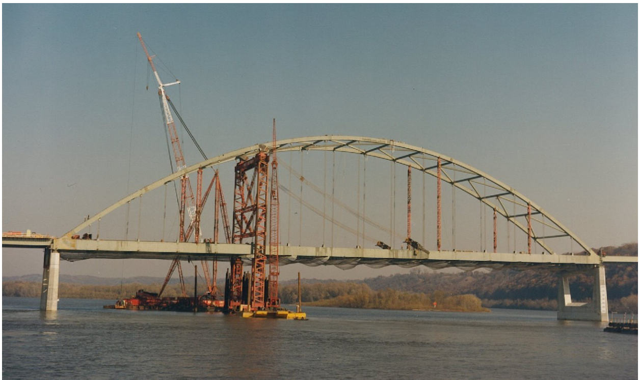
Figure 13 Arch Erection with Falsework
