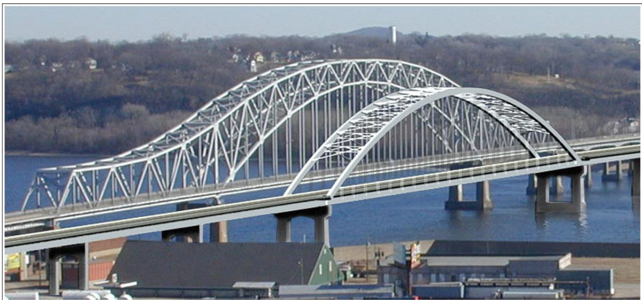
Figure 1: New and Existing U.S. 20 Main Span Bridges
