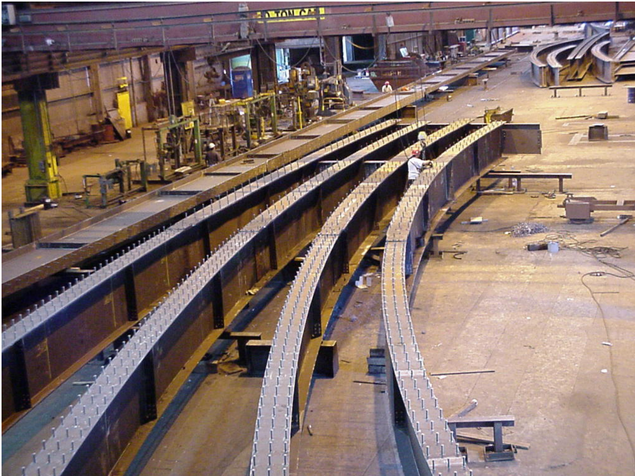
Figure 13: Shop Fit-Up of Non-Concentric Framing
