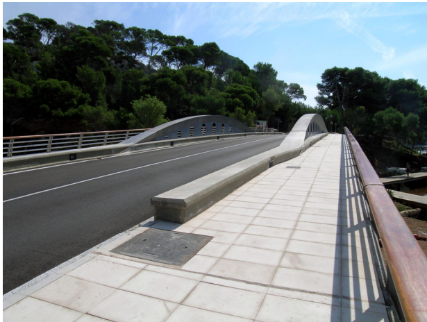
Figure 14. View of the deck.
