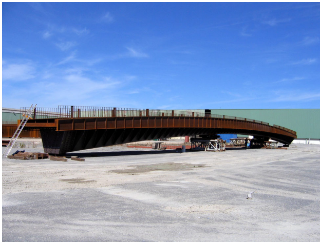
Figure 8. Assembly verification of steel beam at steel yard.
