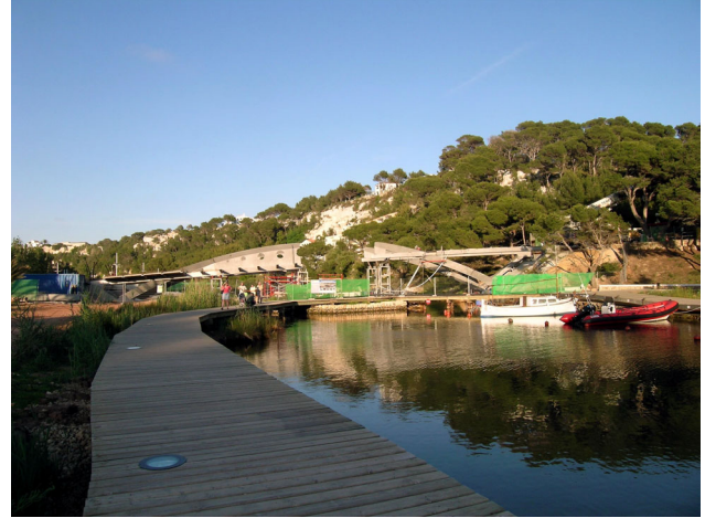
Figure 18. Assembly of the bridge.
