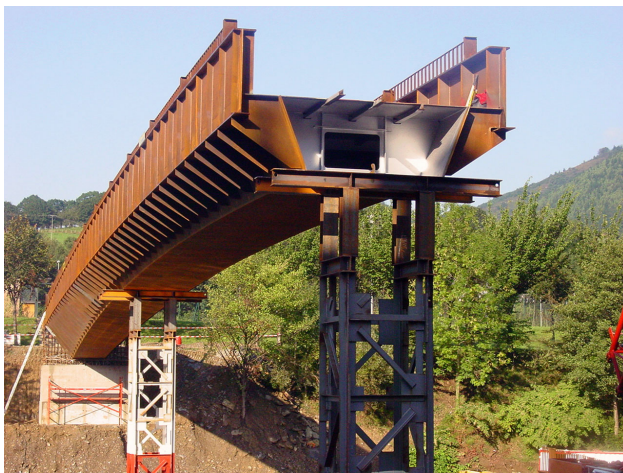
Figure 9. Erection of steel beam.
