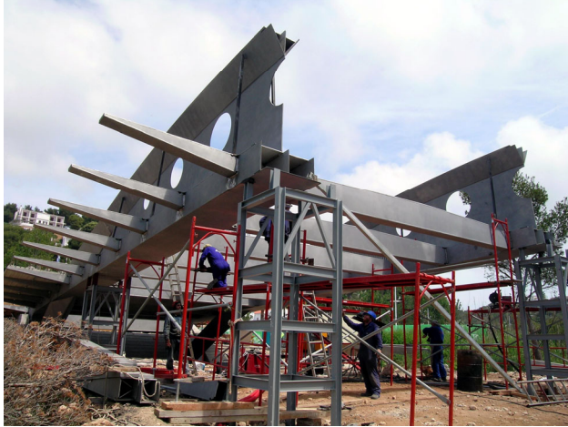
Figure 17. Assembly of the steel structure on temporary supports.
