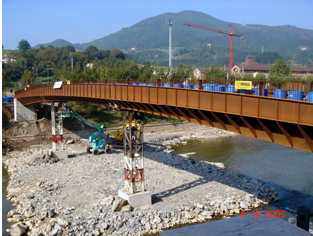
Figure 7. View of the static load test using water containers.
