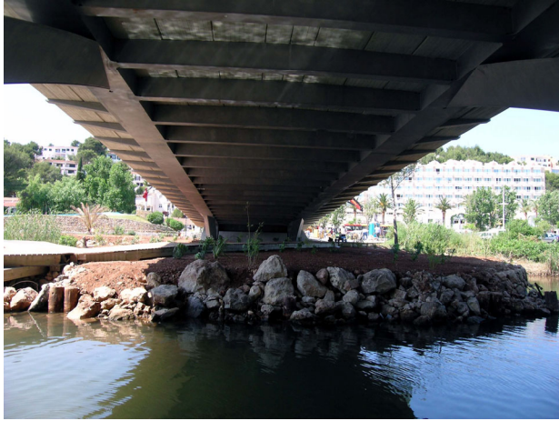
Figure 13. General view of the bridge
