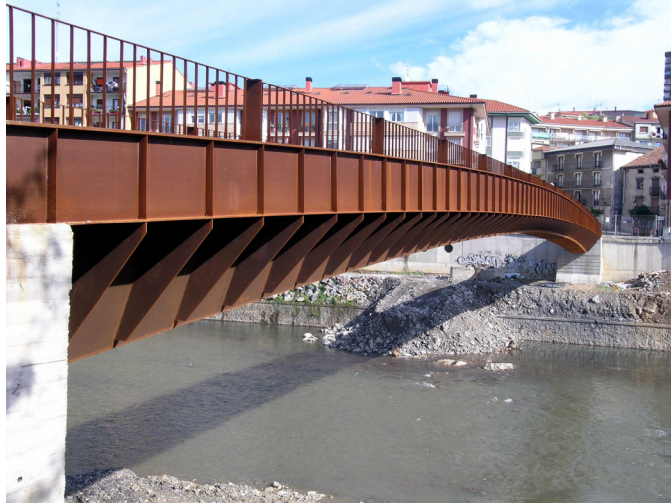
Figure 1. Final view of the footbridge.
