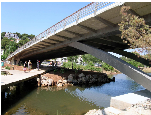
Figure 12. View of the bridge from below
