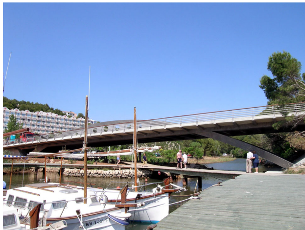
Figure 10. General view of the bridge over Algendar River.
