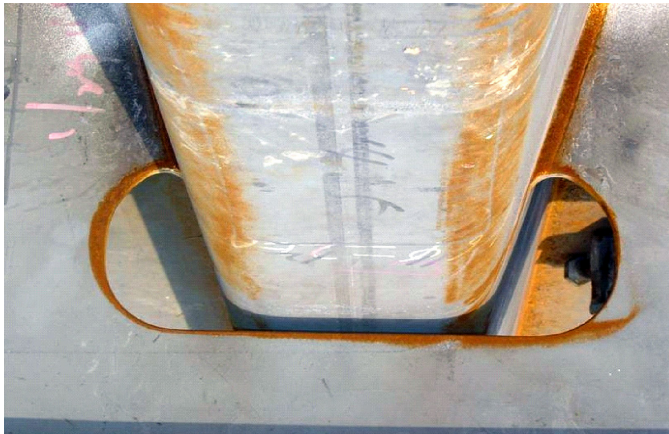
Figure 10: Rib Detail at Diaphragm
