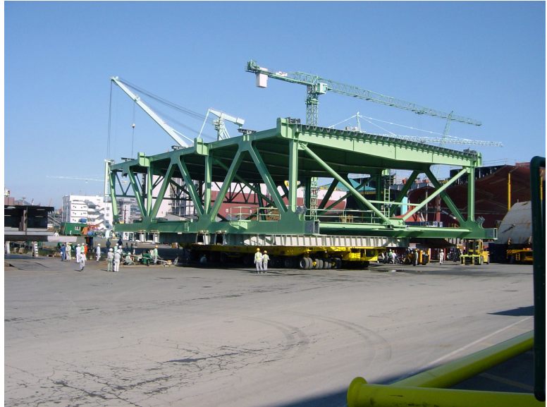
Figure 12: Completed Bridge Segment (TNC)
