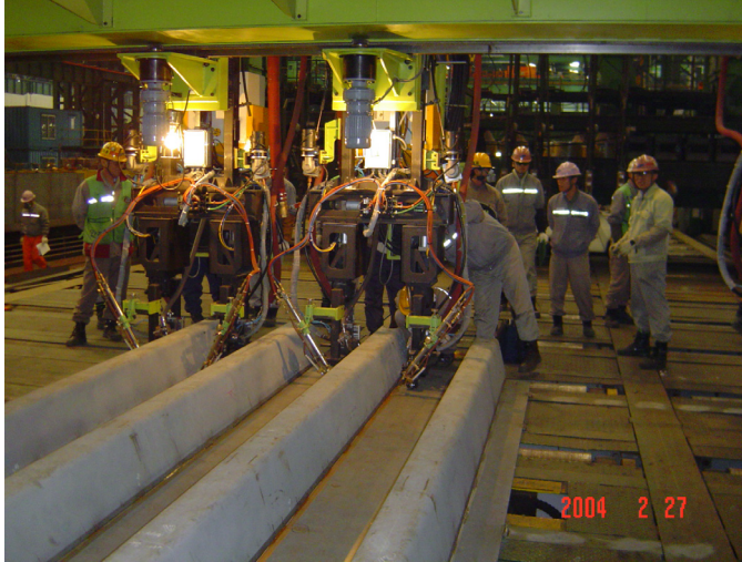
Figure 9: SAW Gantry Welding
