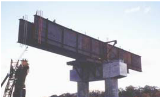
Fig. 9 – Pier Brackets
