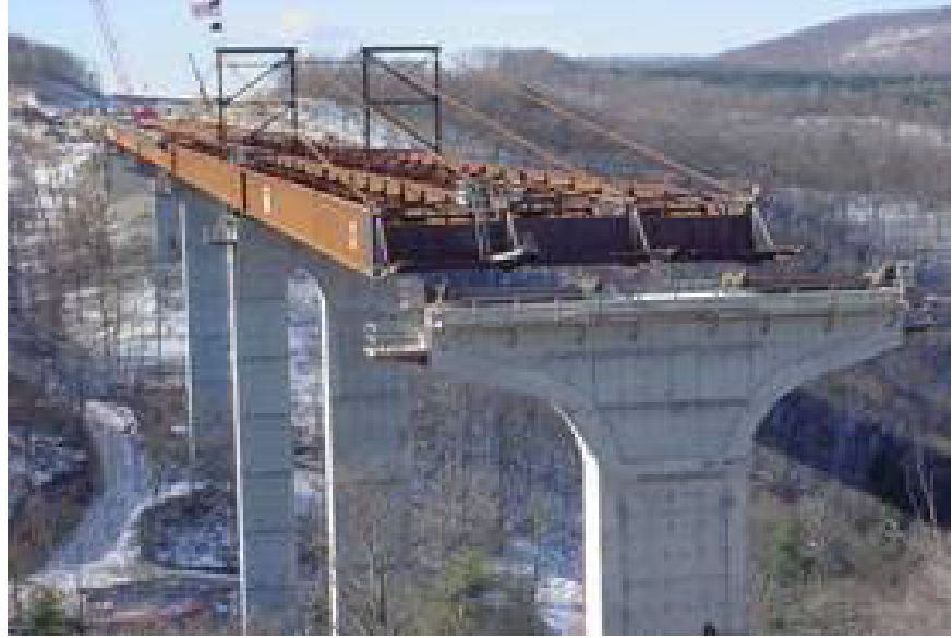
Fig. 11 – I-girder Launch with Cable Tie-Backs
