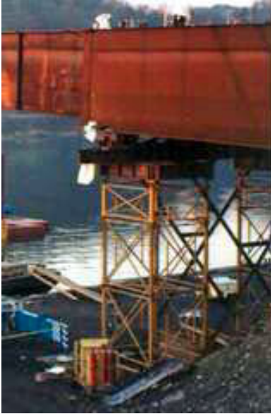
Fig. 10 – Temporary Bent
