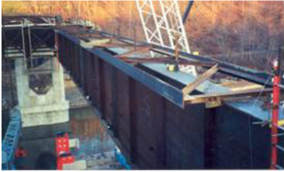
Fig. 7 – Temporary Top Flange Stiffening Truss
