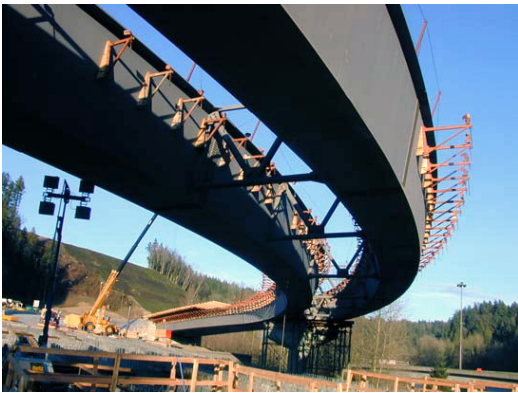
Figure 11: The Girders Erected
