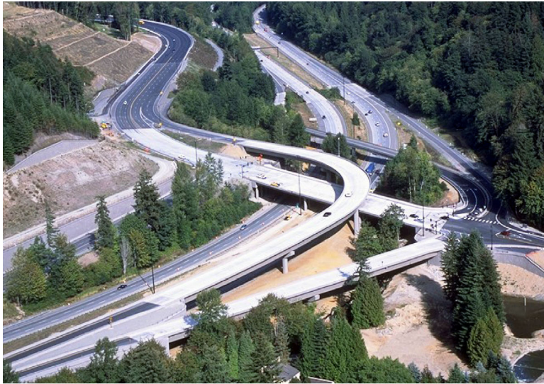
Figure 1: the I-90 Sunset Interchange
