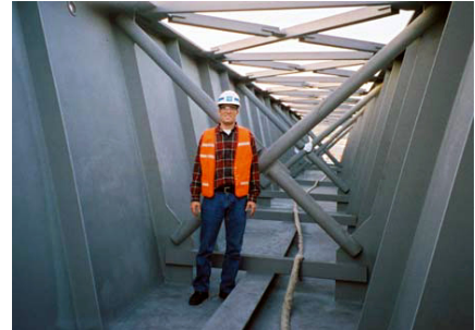
Figure 13: Cross Frames and Lateral Bracings inside the steel box girder
