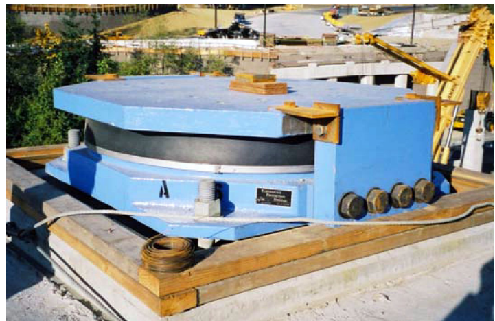
Figure 22: Friction Pendulum Bearings in Place
