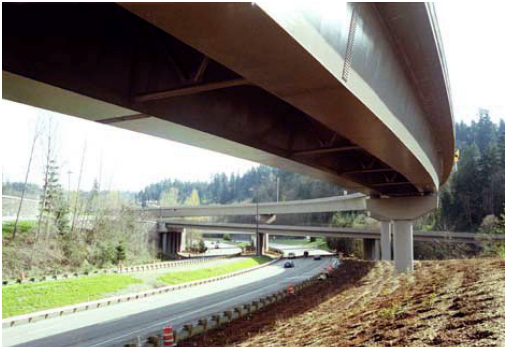
Figure 28: Flyover Bridge Looking East
