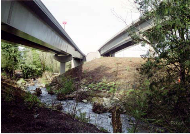
Figure 29: Flyover Bridge and Issaquah Crossing Bridge Looking West
