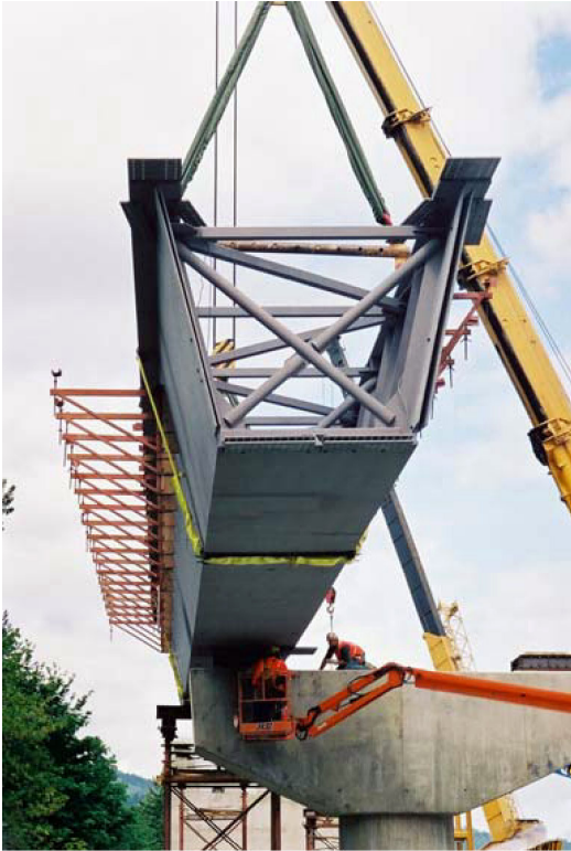
Figure 9: Steel Box Girder Erection
