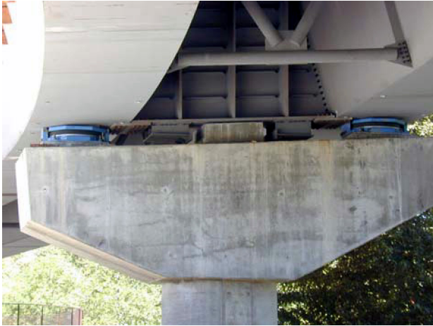
Figure 16: Isolation Bearings under Girders
