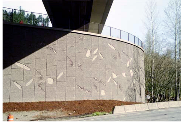
Figure 30: Retaining Wall with Floral Leaf Imprints under the Flyover Bridge
