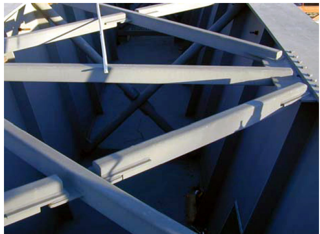
Figure 15: Tubing Sealed for Corrosion Protection
