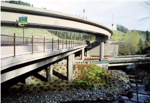
Figure 27: Flyover Bridge (Top) Looking
