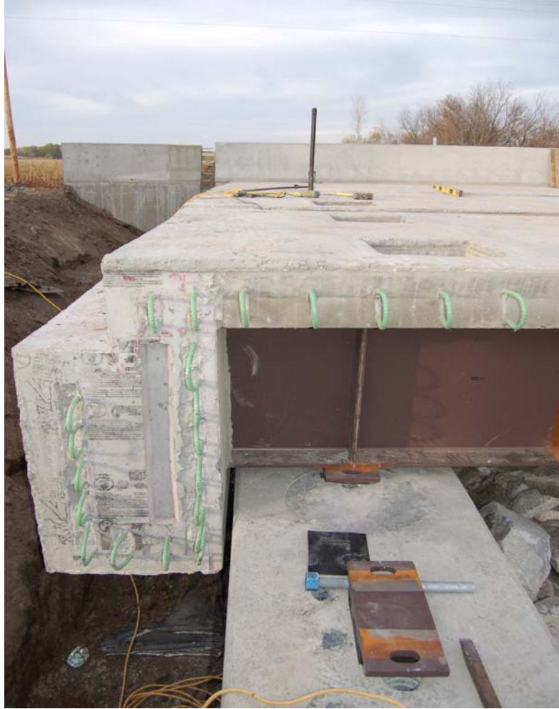
Figure 7. End span module with suspended backwall
