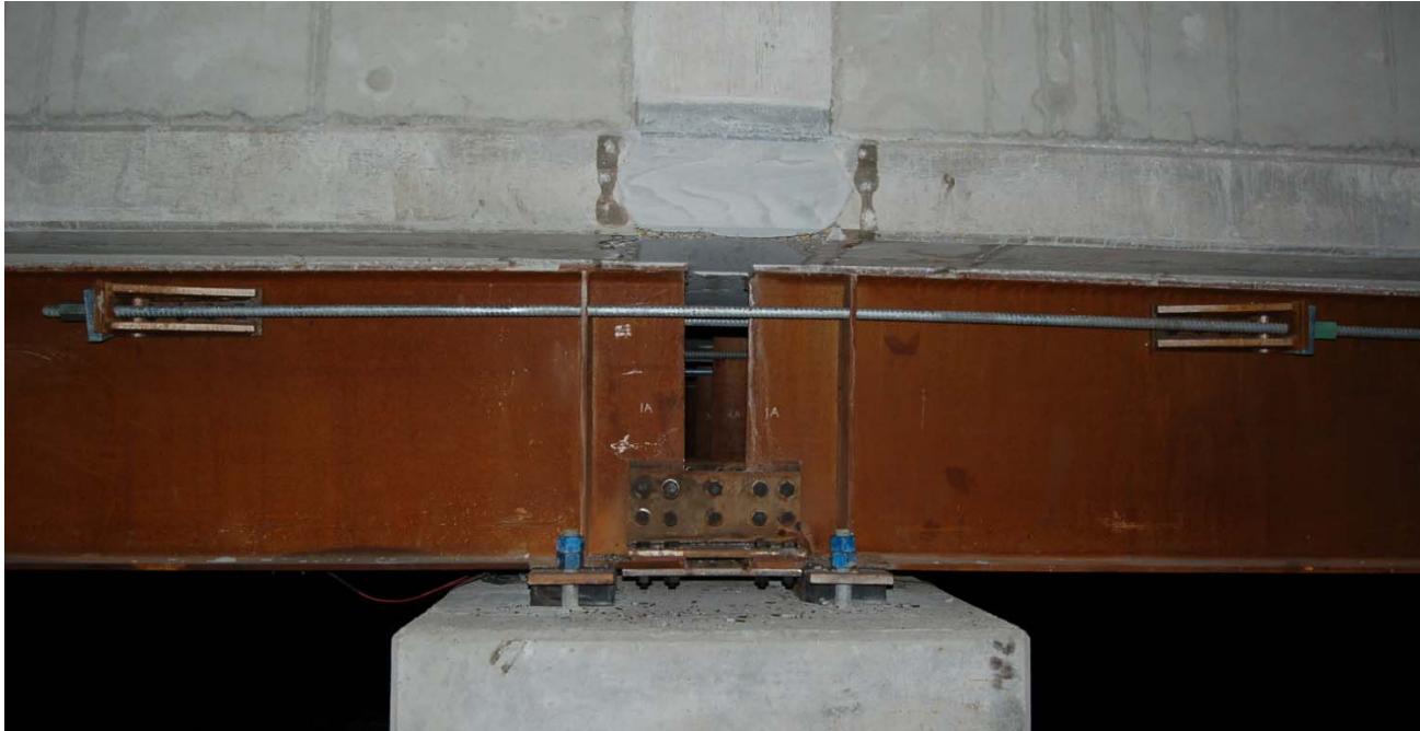
Figure 11. Post-tensioned retrofit for modules
