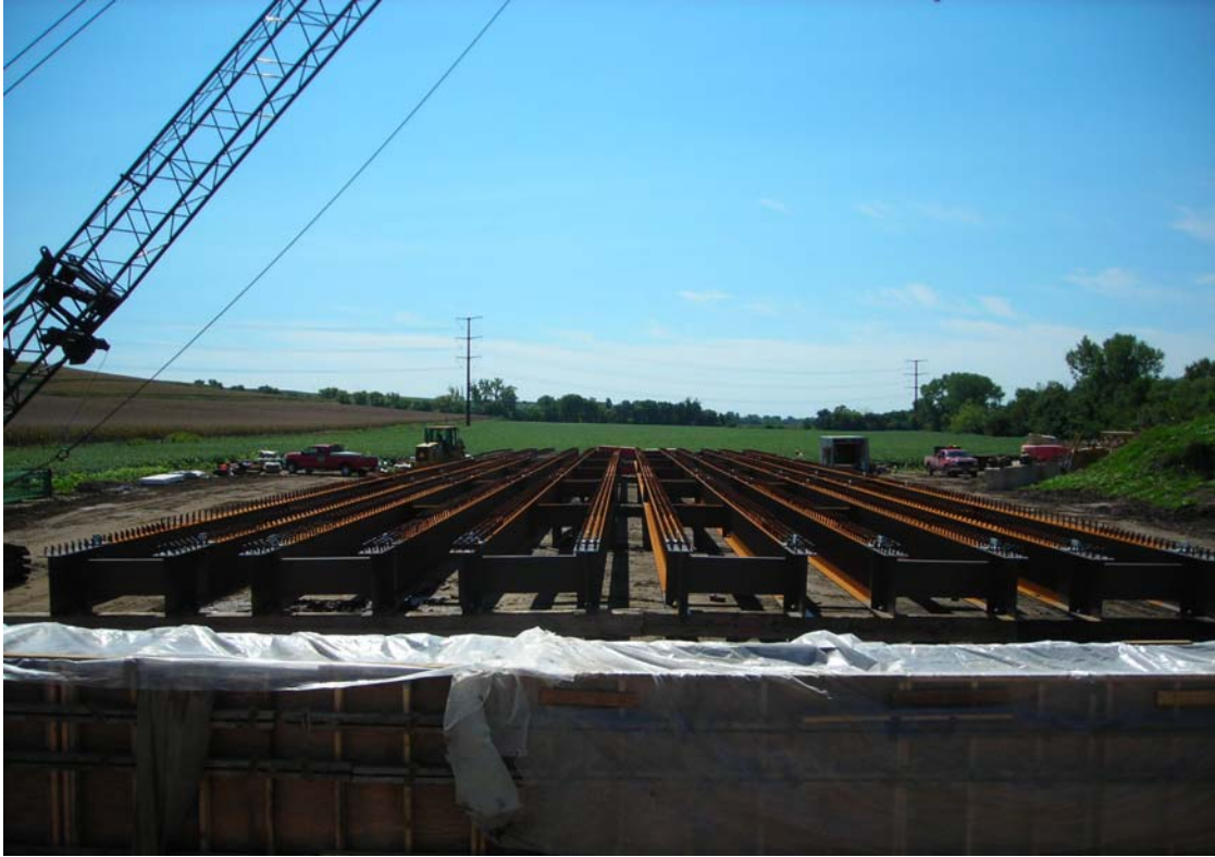
Figure 6. Timber falsework bents for module assembly
