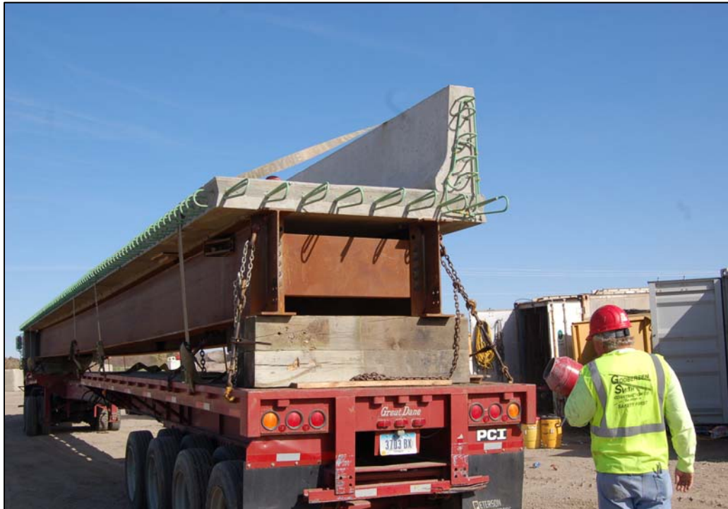
Figure 4. Exterior superstructure module during shipment to bridge site
