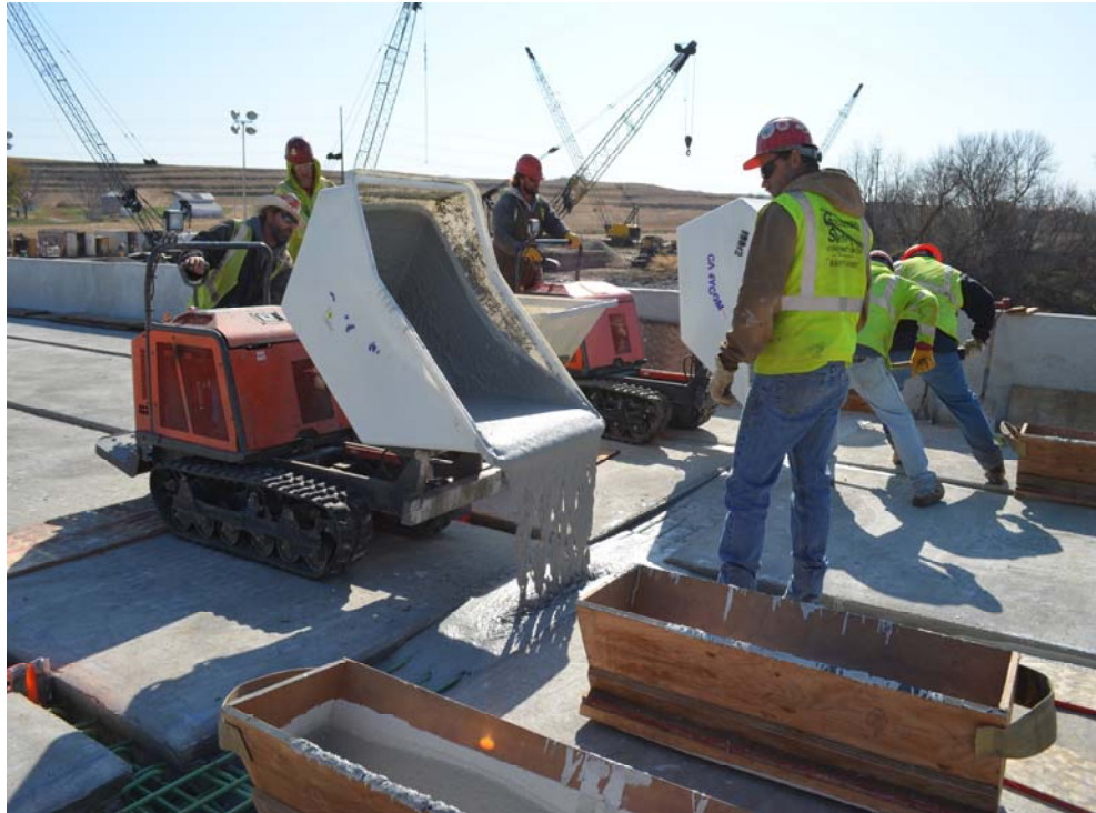
Figure 8. Placement of UHPC concrete for superstructure joints.
