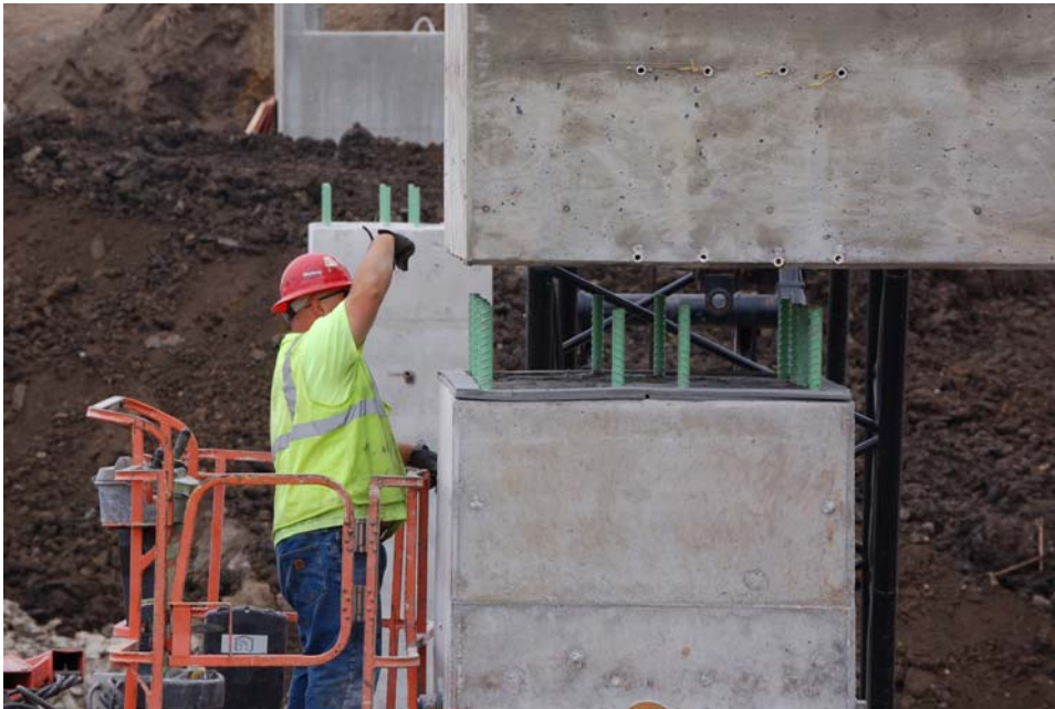
Figure 9. Connection of precast cap to precast column
