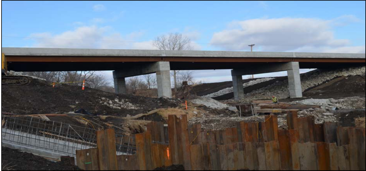
Figure 2. Completed ABC Demonstration Bridge
