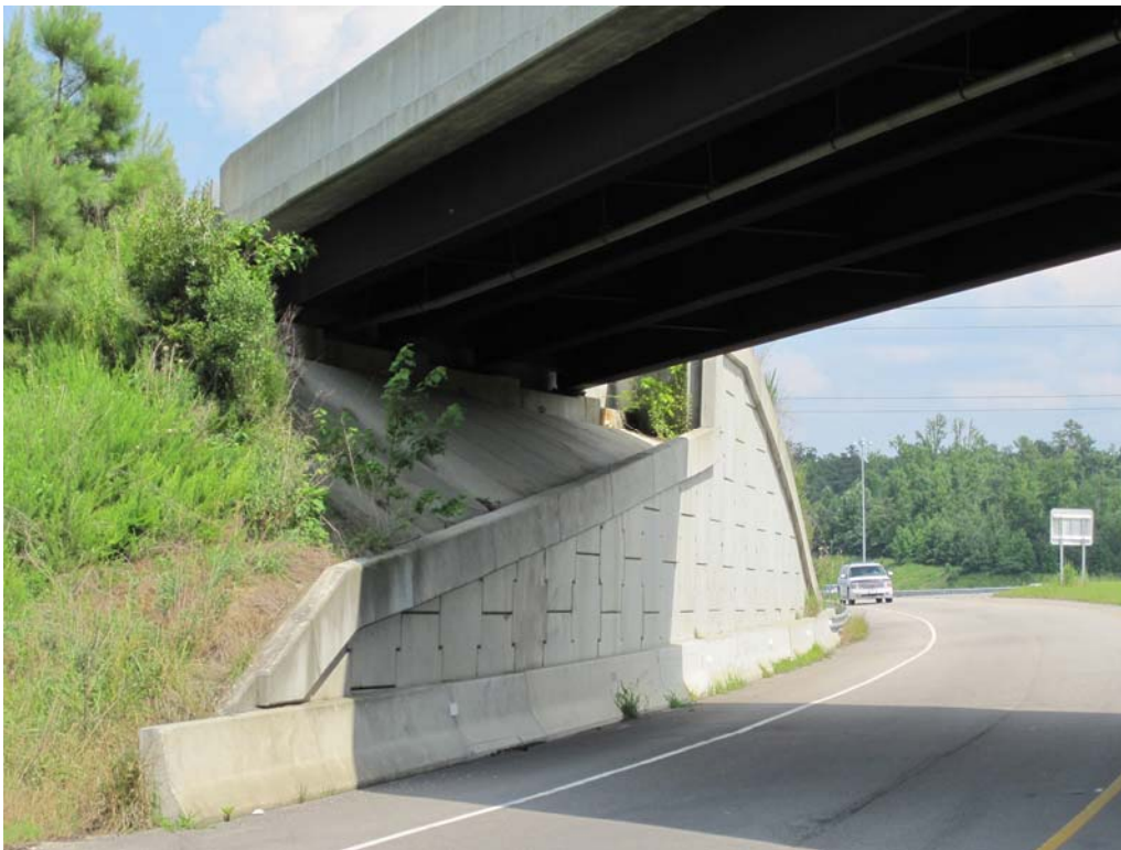
Figure 9: A steel girder bridge where a small mechanically stabilized earth (MSE) retaining wall was used to reduce the severity of skew without significant increase in span length.
