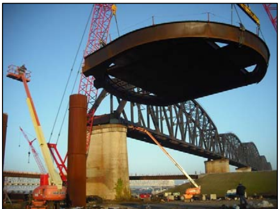
Figure 5 - Lifting of Assembled Platform
