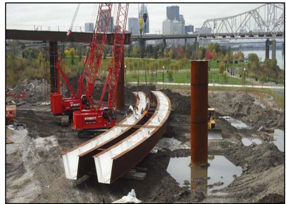
Figure 2 - Ramp Girder Cross-Section during Assembly
