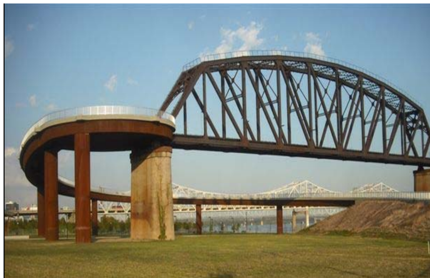
Figure 7 - Completed Pedestrian Ramp
