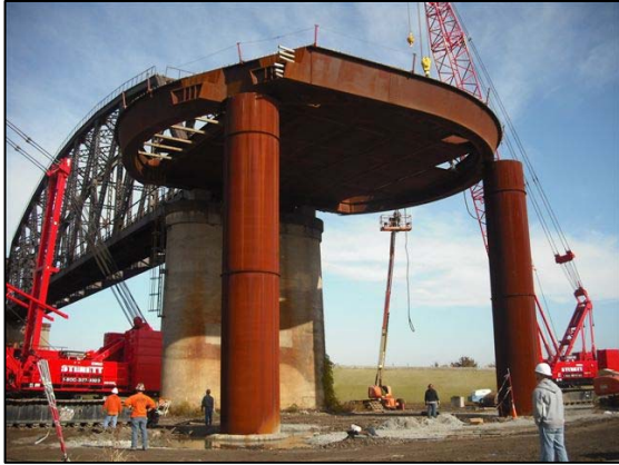
Figure 6 - Platform Assembled and Placed
