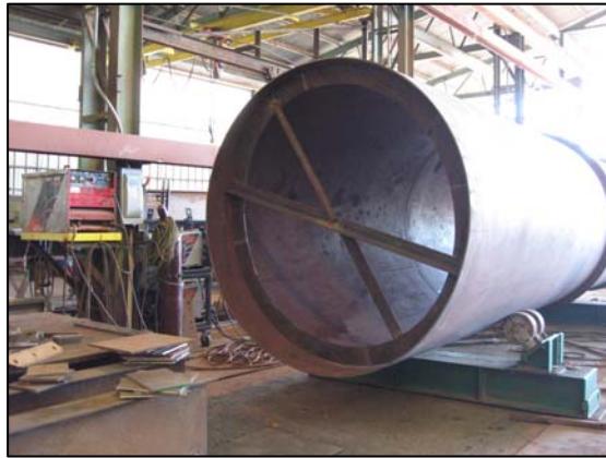
Figure 4 - Steel Pier Shell/Form
