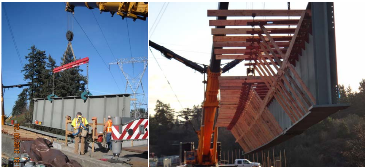
Figure 5 ~ Girder Erection
