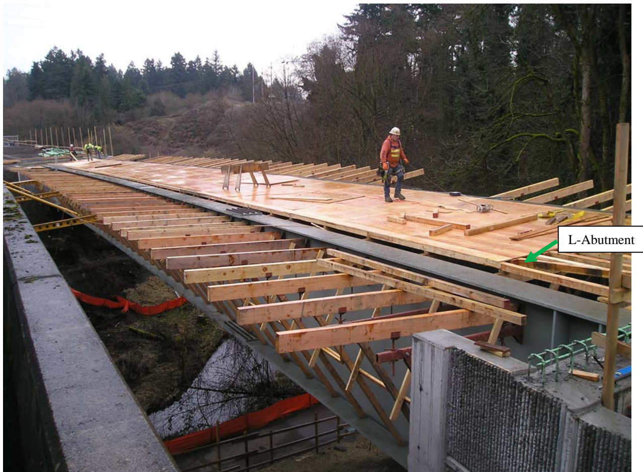
Figure 7 ~ SE Bridge Project as of February 2012
