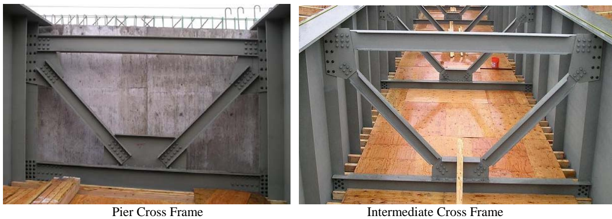
Figure 4 ~ Cross Frame Designs
