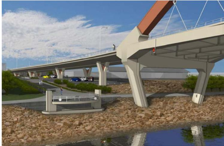
Figure 3 – Framed Knuckle and Integral Pier
