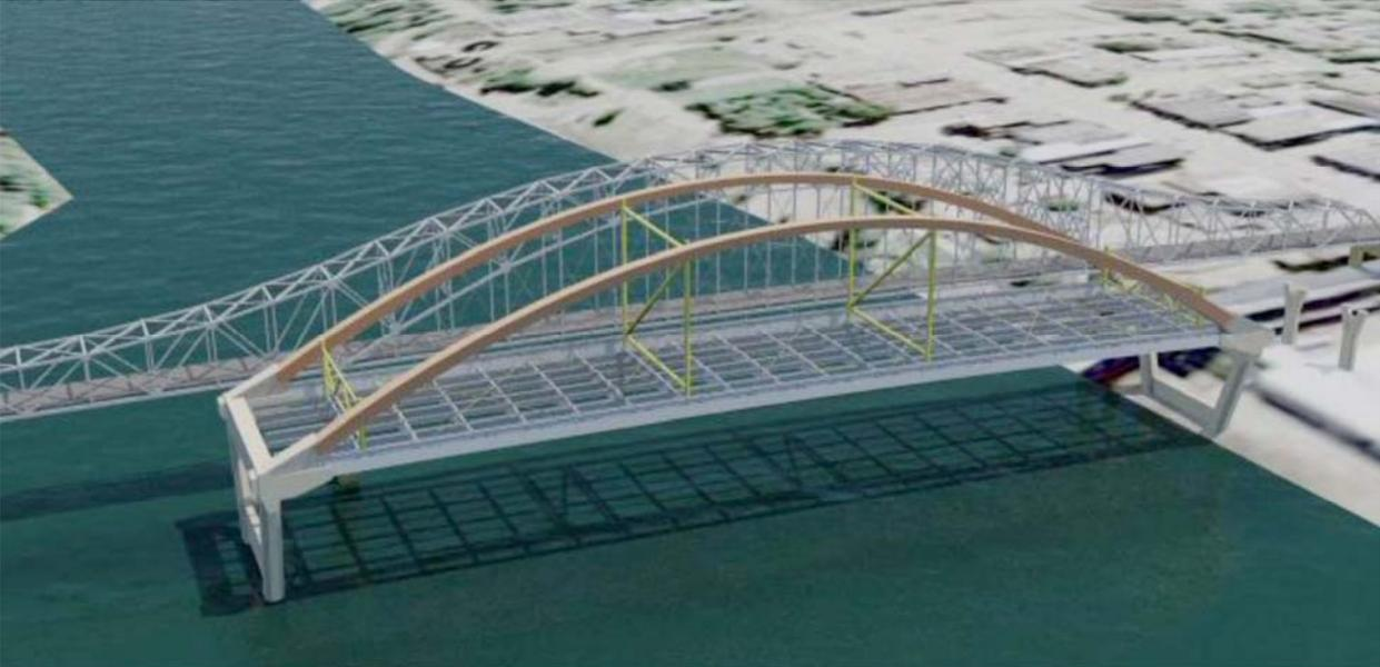
Figure 18 – Knuckle and Tie Girder Placement
