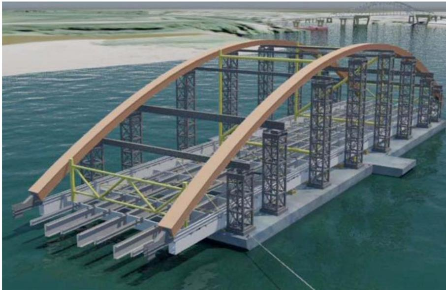
Figure 15 – Arch Erection with Temporary Towers
