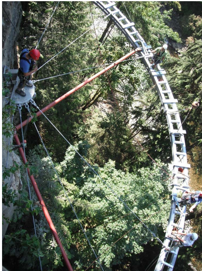
Figure 11. Temporary bracing members (red) for the construction of the curved bridge.
