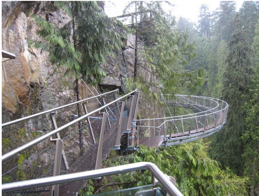
Figure 1. Cliffwalk general view.
