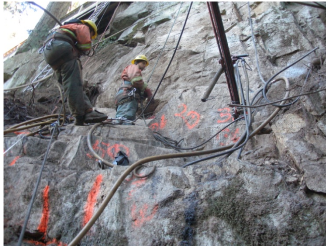
Figure 5. Typical rock bolting construction.
