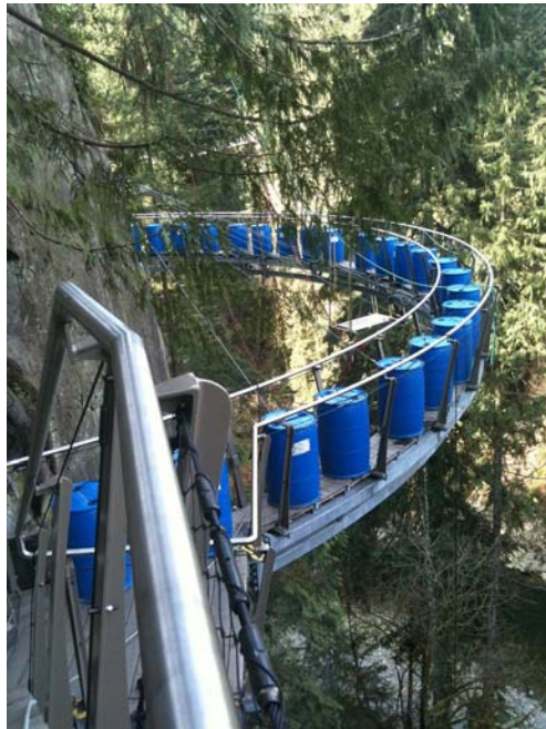
Figure 13. Load testing the curved bridge with water barrels.
