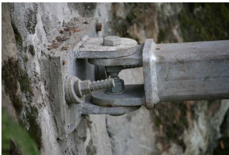
Figure 6. Strut beam plate and rock anchors.
