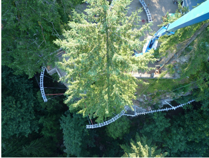
Figure 12. Erection of the curved bridge.
