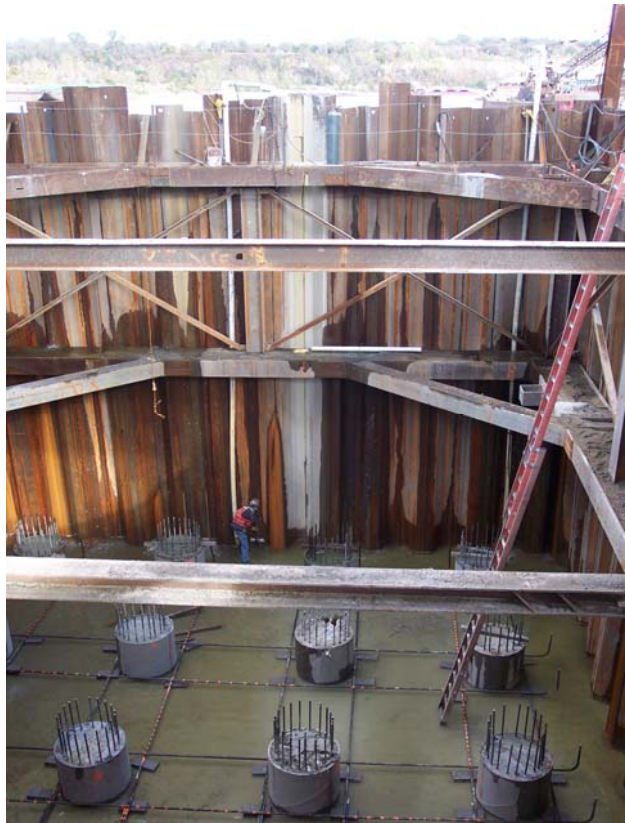
Figure 5 - River piers utilized 42-inch steel shell piles constructed inside deep
