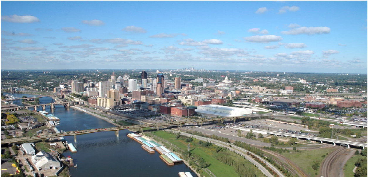
Figure 1 - Rendering of final bridge against the City of St. Paul with the Minneapolis skyline in the background.
