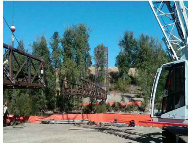
Figure 7 Setting truss sections
