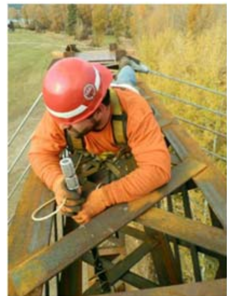
Figure 8 Testing tower bolt torques
