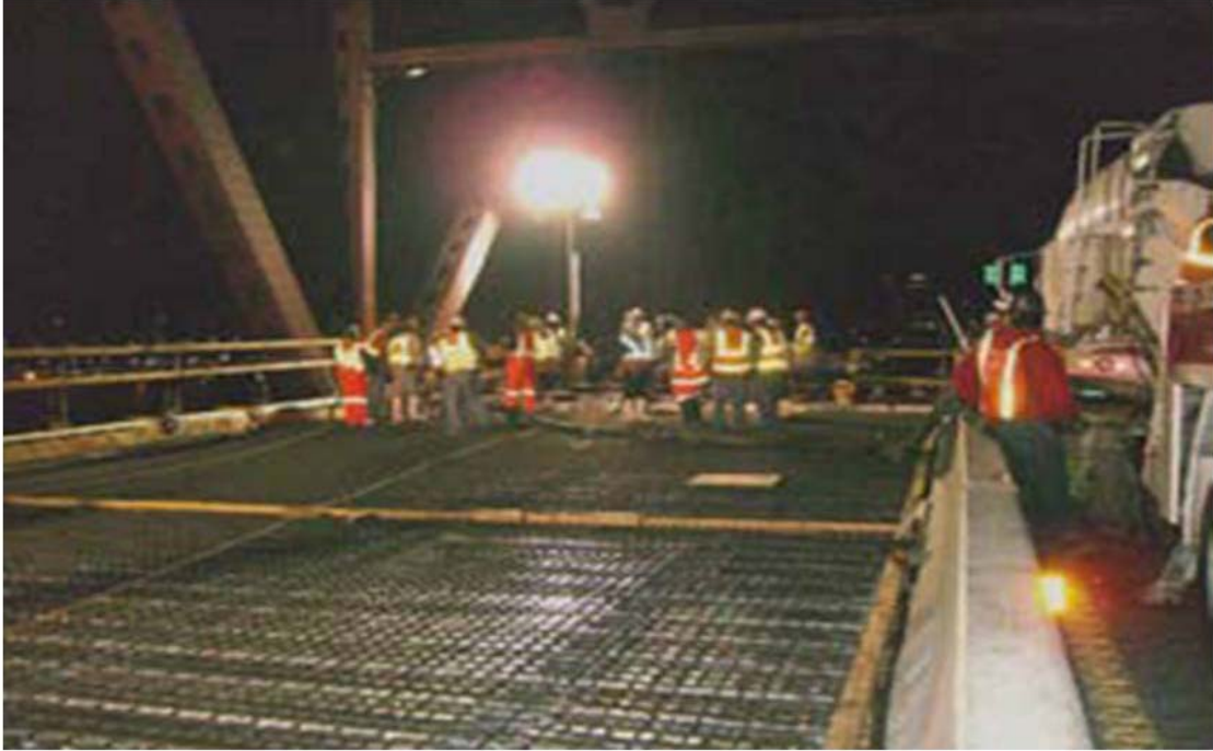
Figure 15: Night-time concrete deck pours.
