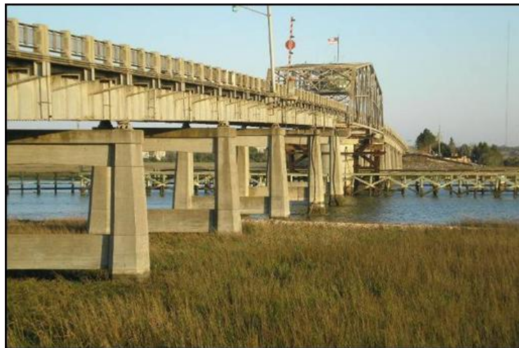
Figure 3: Ben Sawyer Bridge prior to the rehabilitation.
