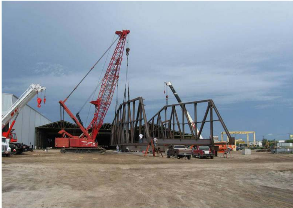
Figure 17: Swing span shop erection at FSS yard.
