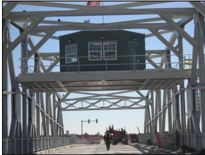
Figure 10: Control House at mid-span above the roadway.
