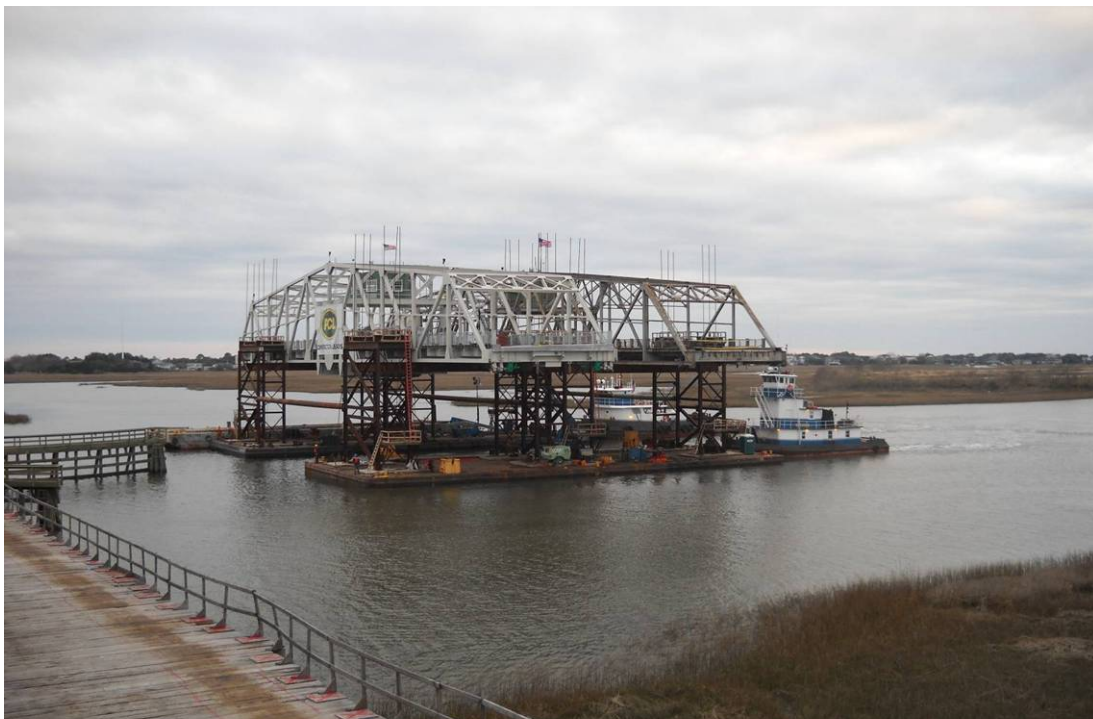
Figure 18: Float-in barges with new and old swing spans.
