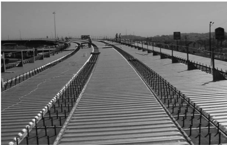
Figure 1. SIP forms in a bridge prior deck placement
