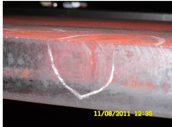
Figure 9. Crack observed after plasma cutting in 1¾” plate.
