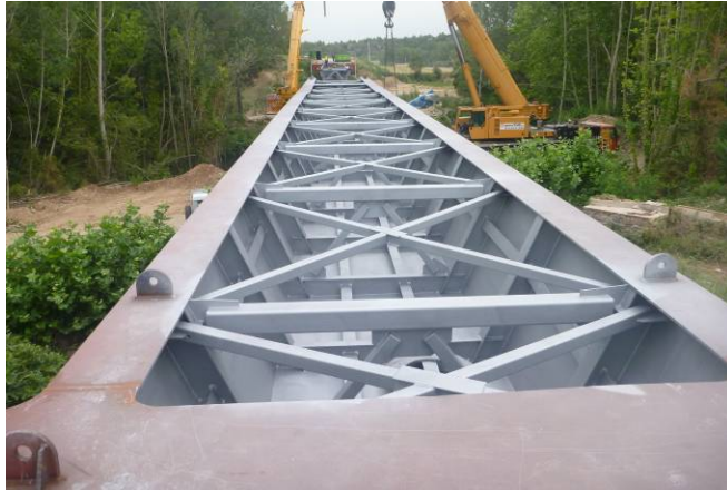
Figure 3-5. Detail of top lateral bracing
