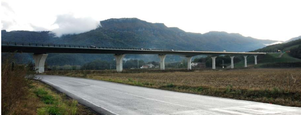
Figure 2-1. Bridge at Vall d'en Bas
