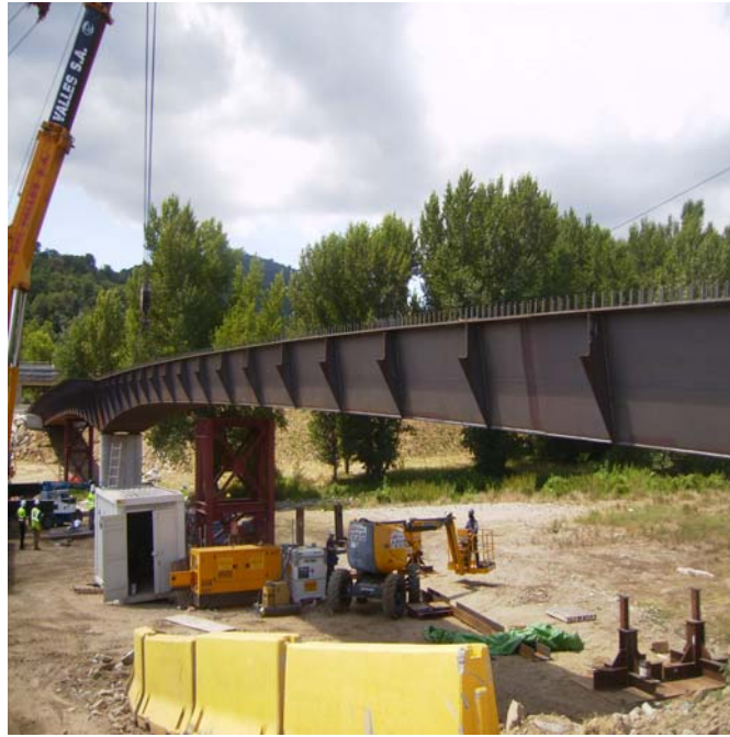
Figure 4-8. Installation of the top slab precast panels.
