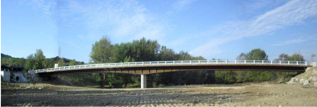
Figure 4-1. Bridge over Tordera River in Sant Celoni.
