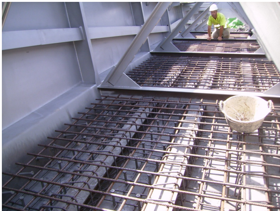
Figure 4-7. Double composite region near intermediate support.
