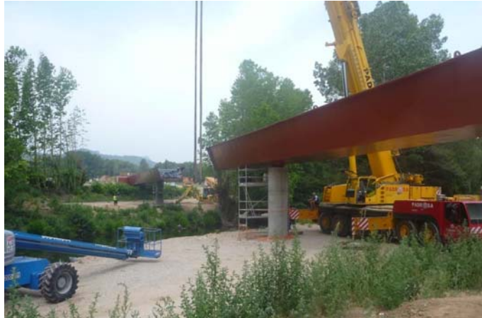
Figure 3-7. Steel girder erection.
