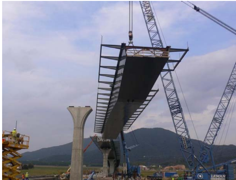
Figure 2-5. Typical section lifted to the final position
