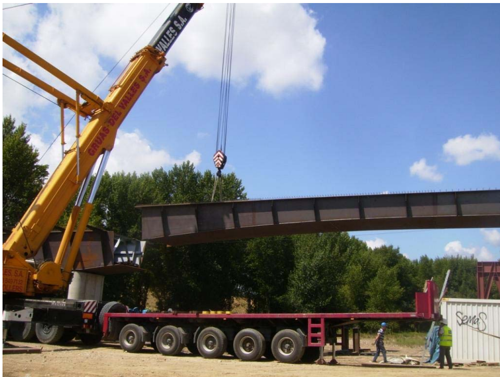
Figure 4-5. Erection of the steel girder.
