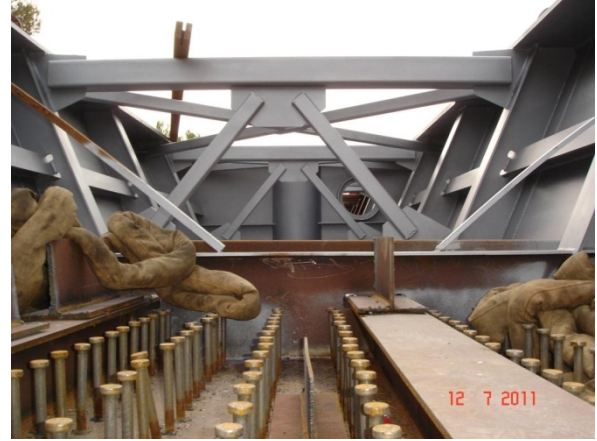
Figure 3-6. Typical and interior diaphragms
