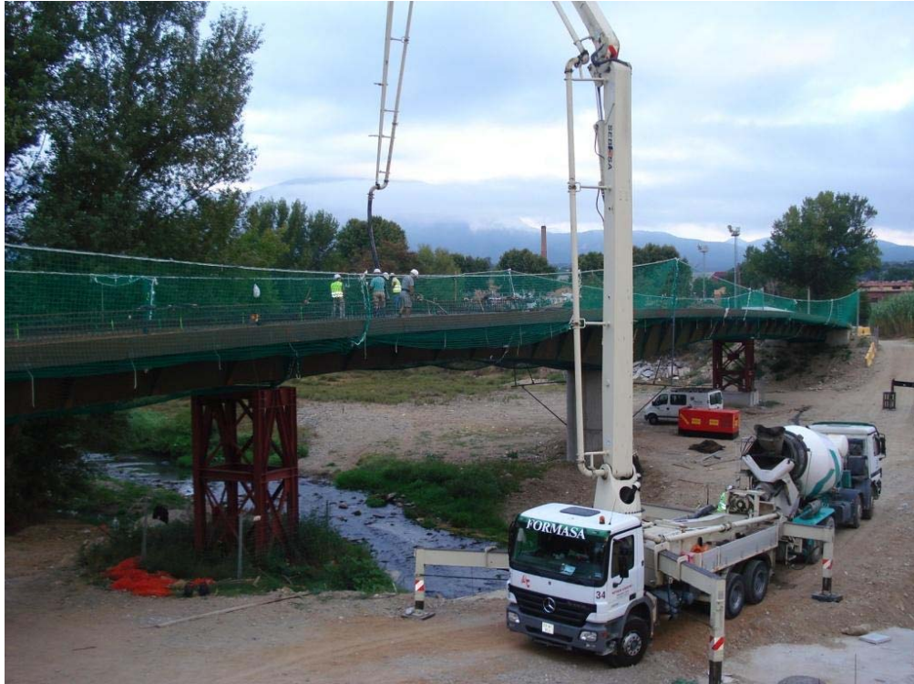
Figure 4-6. Steel girder on temporary supports.
