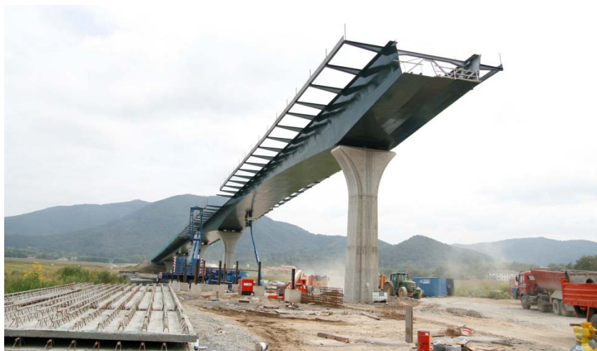
Figure 2-6. Installation of the steel girder and precast panels
