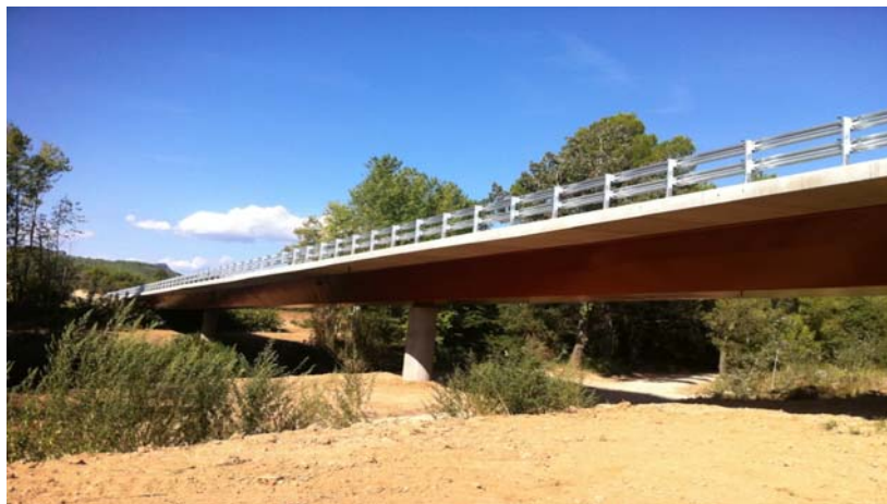
Figure 3-1. Bridge over La Muga River at Les Escaules (Girona, Spain)
