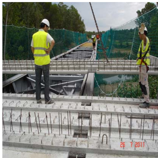
Figure 3-8. Precast concrete panels of the top slab.
