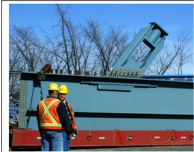
Figure 12 - Stay Anchor Connection to Edge Girder
