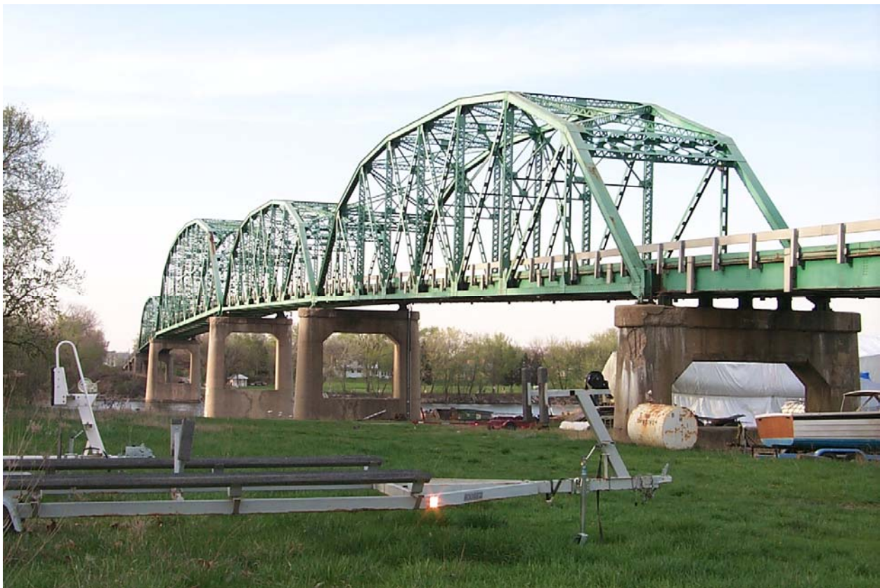
Figure 1: Existing IL-170 Bridge over the Illinois River (Seneca, IL)
