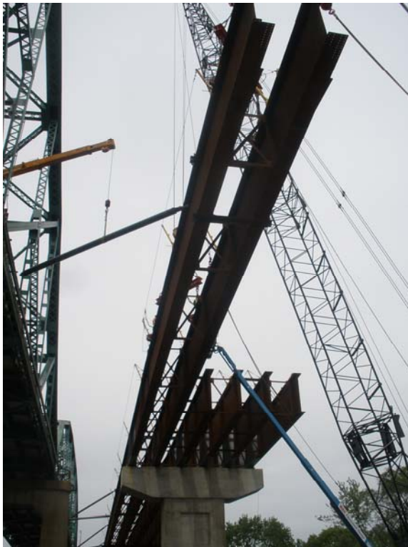
Figure 12: Cantilevered Erection of 2-Girders with External Pipe Bracing to Existing Truss
