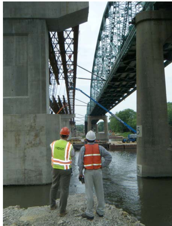
Figure 13: Drop-in Erection of Gate Segment with External Pipe Bracing to Existing Truss
