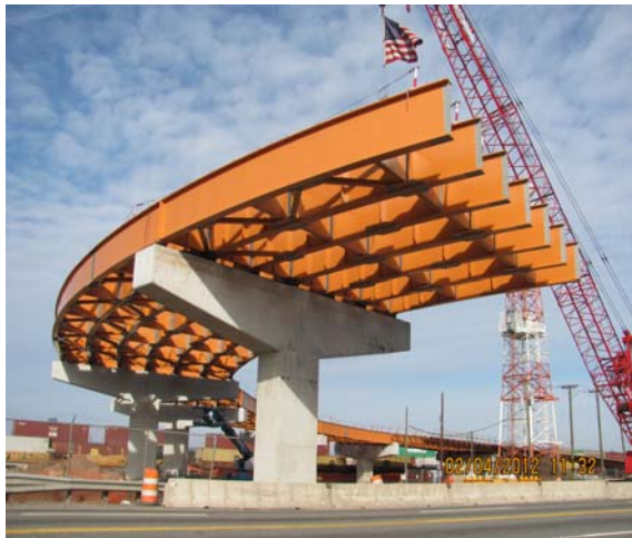
Figure 5: Photo of erected curved girders
