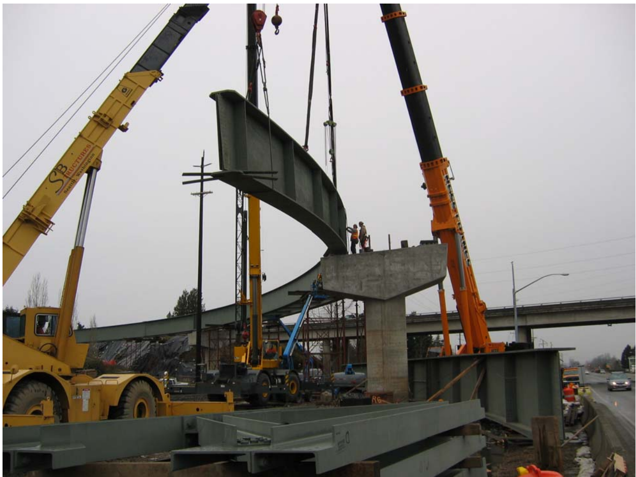
Figure 8 Two Cranes Held the Curve Girder during Erection
