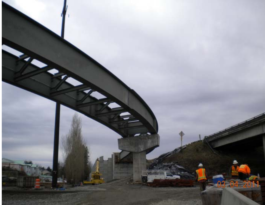
Figure 6 Bridge Construction Site
