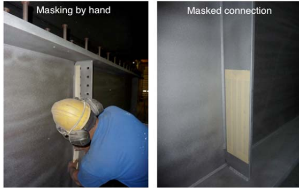
Figure 1: Masking of connection faying surfaces (courtesy of Structural-Bridges, Québec)
