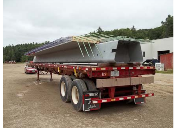
Figure 6. Pre-top folded plate girder
