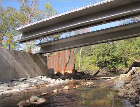
Figure 13. Construction of First Folded Plate Bridge
