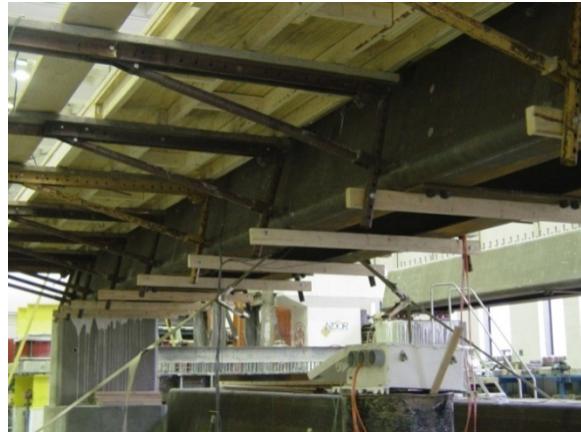
Figure 4. Conventional formwork for casting concrete deck
