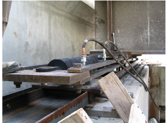
Figure 8: Lateral Slide Push-Pull Jacking System
