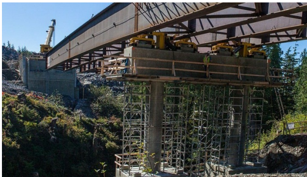
Figure 12: Hilman Rollers and Lateral Guides
