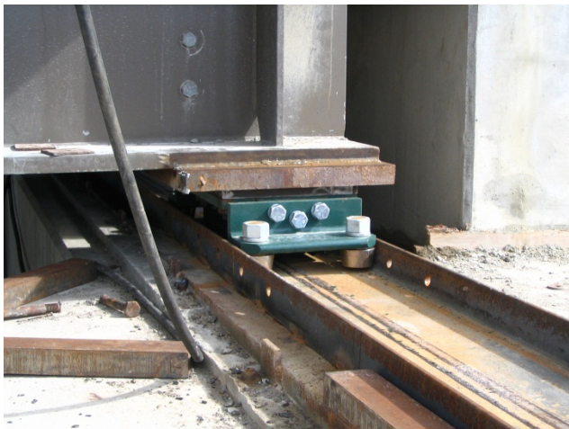
Figure 7: Slide Path with Guided Hilman Rollers
