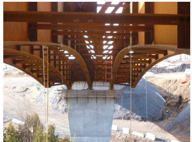
Figure 2: Three Girders Bearing on Pier
