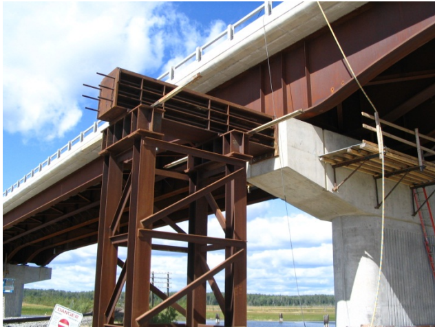
Figure 6: Temporary Bents for Kenogami
