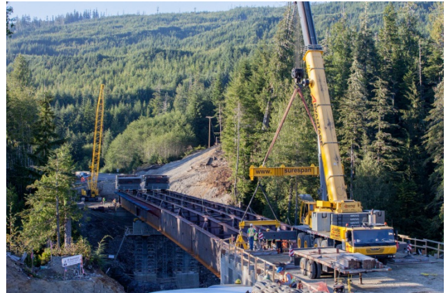
Figure 13: Crane Lift to in Place of Launch Nose
