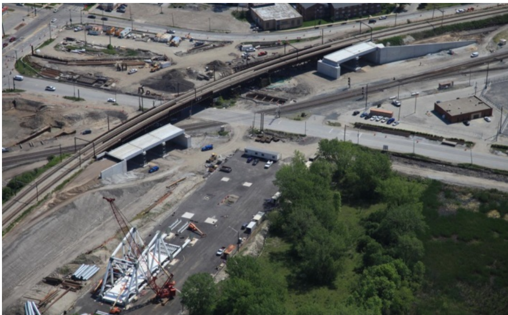
Figure 19: May 2012 - Truss Assembly Begins; Approach Spans in Place
