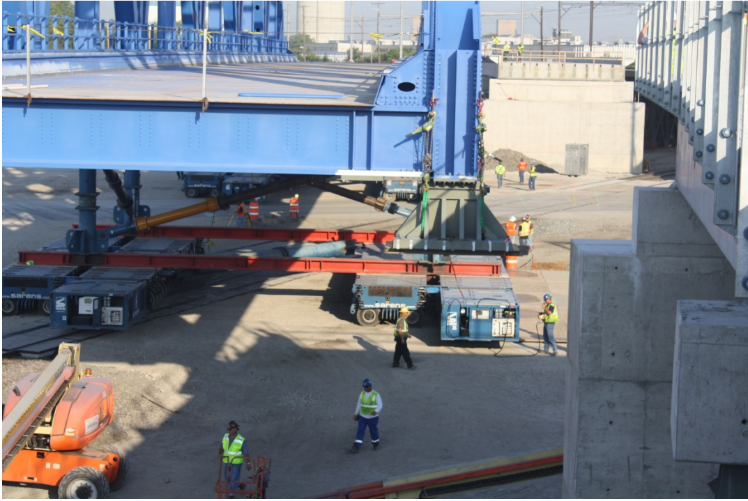
Figure 28: SPMTs move truss towards its foundations (Mega Piers)
