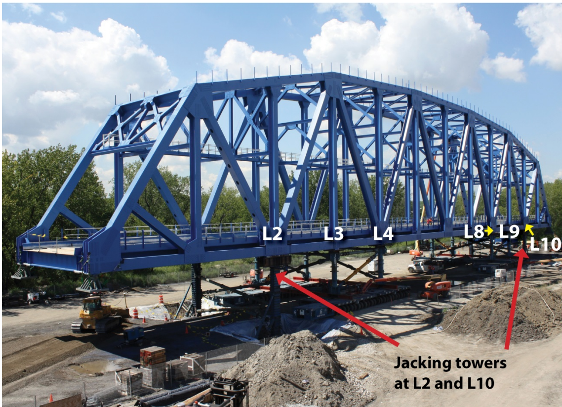
Figure 24: SPMTs at L3 and L4 and at L8 and L9
