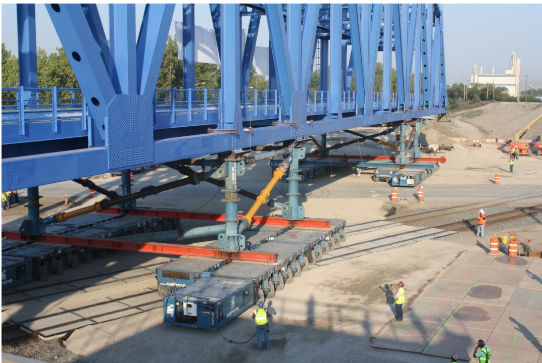
Figure 27: SPMTs moving truss over the existing NS tracks
