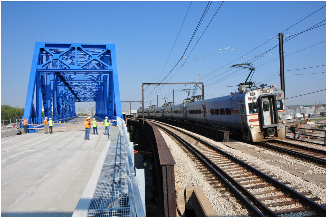
Figure 29: New truss alongside the existing bridge allowing commuter rail service to continue during assembly and installation of truss
