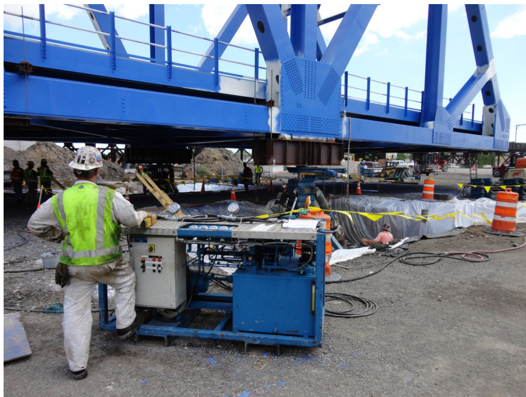
Figure 23: One of the two operators controlling the hydraulic jack operations
