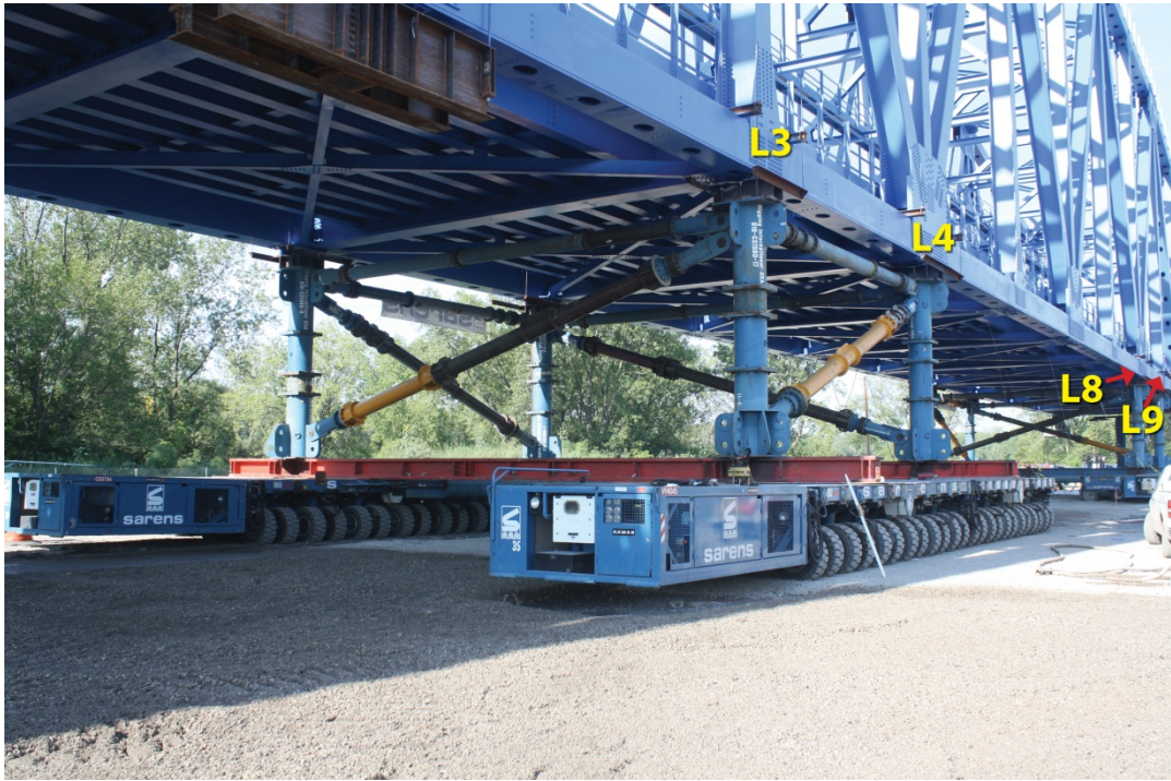
Figure 26: SPMT at L3 and L4 and at L8 and L9
