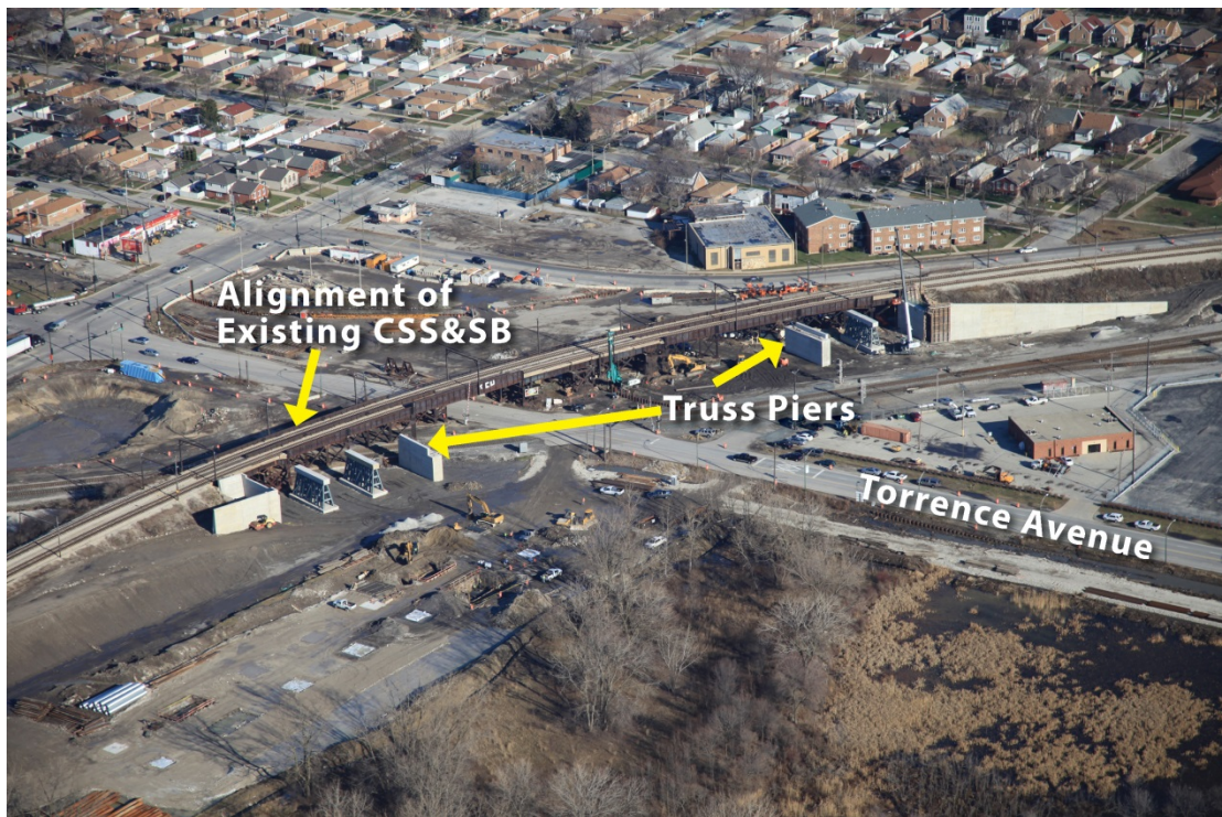
Figure 18: December 2011 - Foundation Units in Place for Truss and Approach
