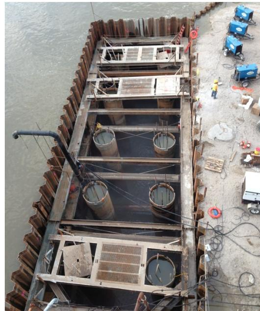
**Figure 4:** Pier 3 Drilled Shaft Construction
