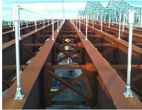
**Figure 8:** Typical Intermediate Cross-frames
