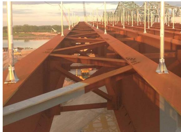
**Figure 9:** Top Flange Lateral Bracing
