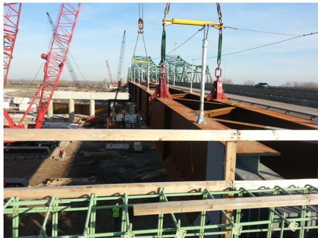
**Figure 15:** Erection of the First Two Girder Pieces in Span 1
