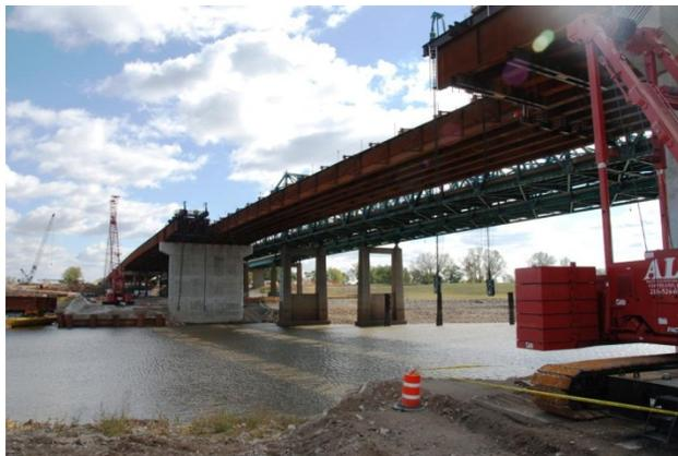
**Figure 16:** Steel Superstructure Prior to the Final Center Span Strand Jack Lift
