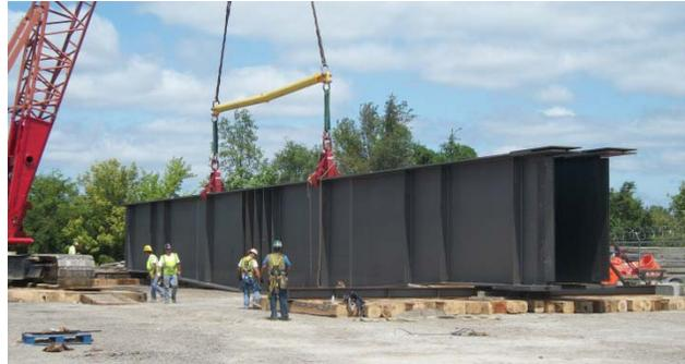
**Figure 14:** Storage of New Bridge Girders in Local Storage Yard
