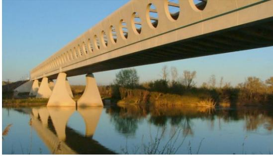
Fig. 7: River Ebro HSR Bridge, designed by CFCSL (2000). The deck is configured as a Vierendeel continuous bridge, built up completely with post-tensioned concrete.
