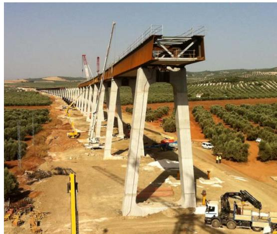
Fig. 9: Archidona Viaduct, designed by IDEAM (2011). 2-mile long composite weathering steel and concrete continuous deck bridge without intermediate expansion joints, designed to extend the composite action to give torsional stiffness to the cross-section in a seismic area (HSR Cordoba-Granada, Spain. See (6)).
