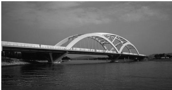
Fig. 8: Garde Adhemar HSR Viaduct in France, designed by Marc Mimram. One of the earliest singular designs using steel for HSR bridges (1995-1999). Note the unusual link connecting the two bowstring arches, necessary to withstand dynamic loading.
