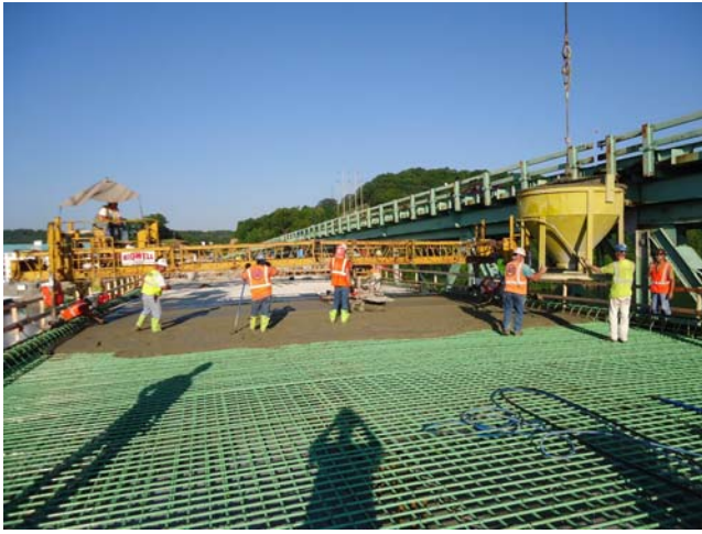
Figure 18 – Concrete Deck Placement
