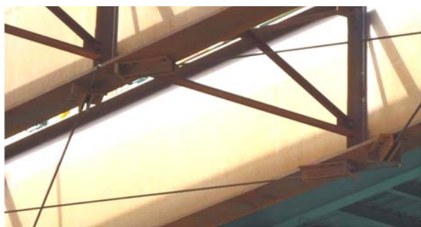
Figure 14 – Lower Lateral Bracing
