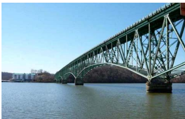
Figure 2 – Existing Hurricane Deck Bridge
