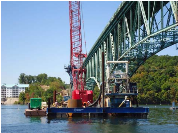
Figure 16 - Worth RCD Drill in Operation
