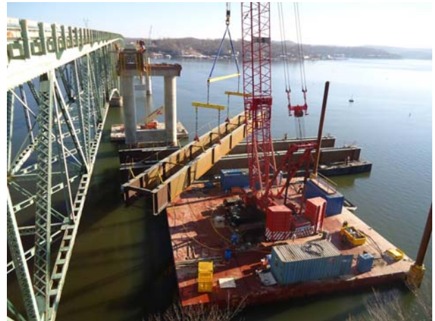
Figure 17 - Girder Erection in Pairs
