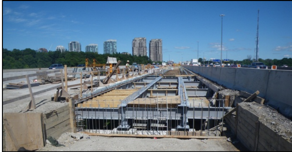
Figure 14: End (Approach) Spans to be constructed in 8 laterally-connected segments
