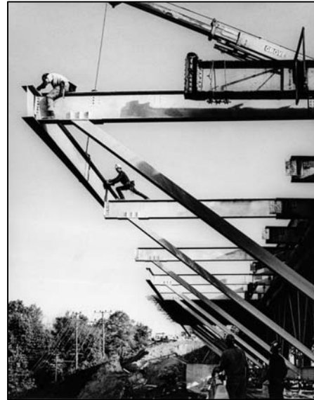
Figure 8: Deck widening of Leaside Truss Bridge in Toronto in the late 1960's
