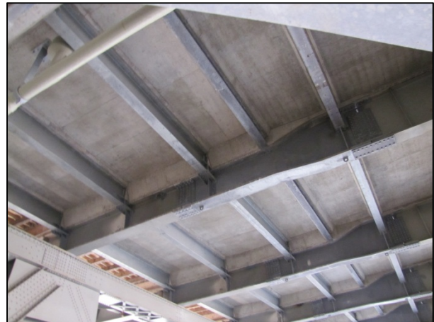
Figure 13: New Stringer System
