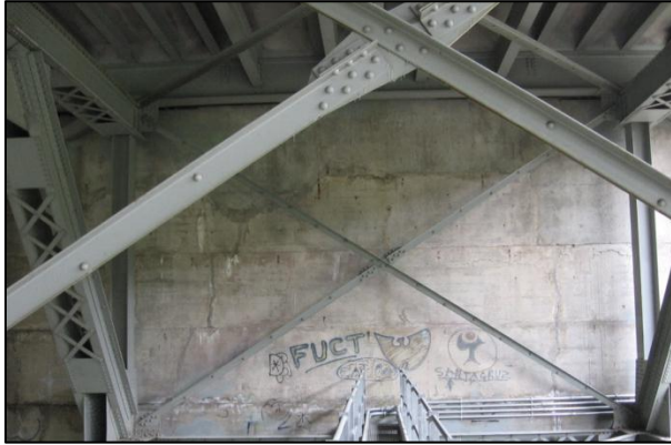
Figure 10: Existing Intermediate Cross Frames
