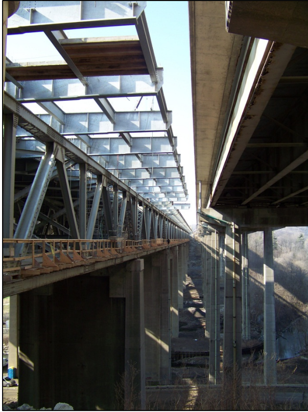
Figure 6: Floor Beam Extension
