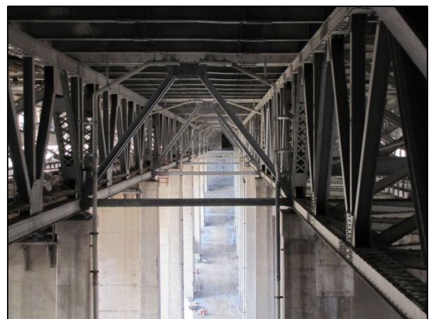
Figure 9: Additional Cross-Frames at Pier Nodes
