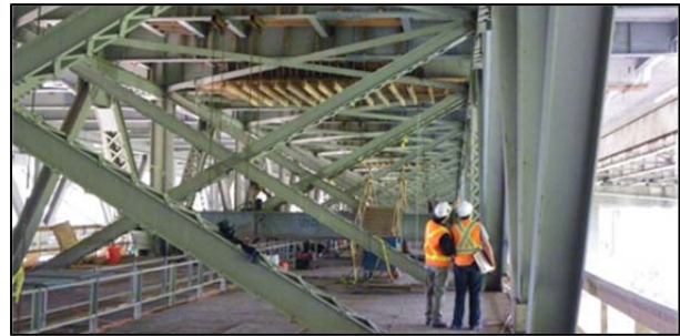
Figure 19: Both Workers and Inspectors can make use of the platforms to access various structural members
