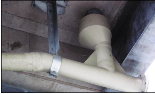
Figure 20: New Deck Drainage System
