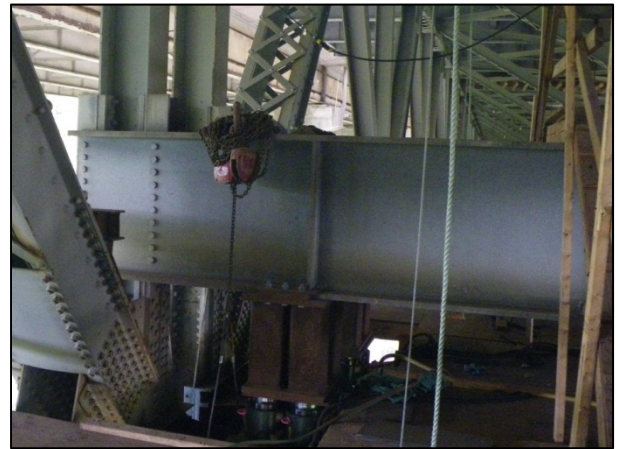
Figure 16: Additional Beam Installed to Facilitate Jacking and Replacement of Bearings
