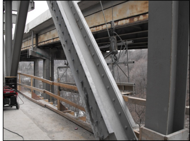
Figure 12: Strengthening of Diagonal Members of Steel Trusses
