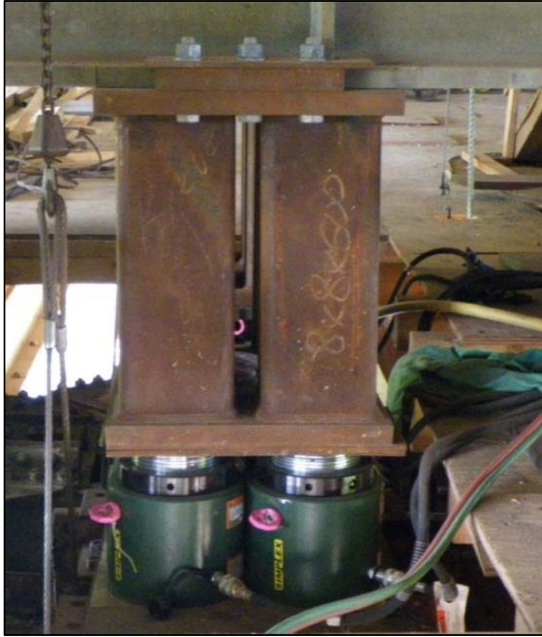
Figure 17: Coordinated Quadruple Jacks at each Bearing Location
