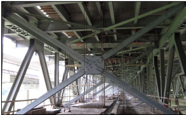
Figure 11: New Intermediate Cross Frames
