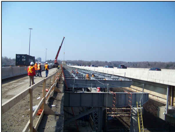
Figure 7: Floor Beam Extension
