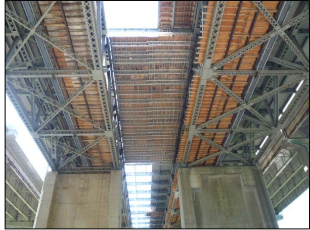
Figure 18: Access Platform at Lower Chord and Spanning Between Trusses
