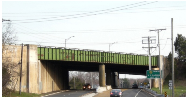
Figure 1. Southbound Garden State Parkway bridge over US Route 9/NJ Route 166.
