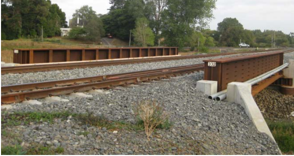
Figure 4: Br 332 NIMT featuring a twin track span 17m long and weighing 95 tonnes. The track centres are 4m apart.
