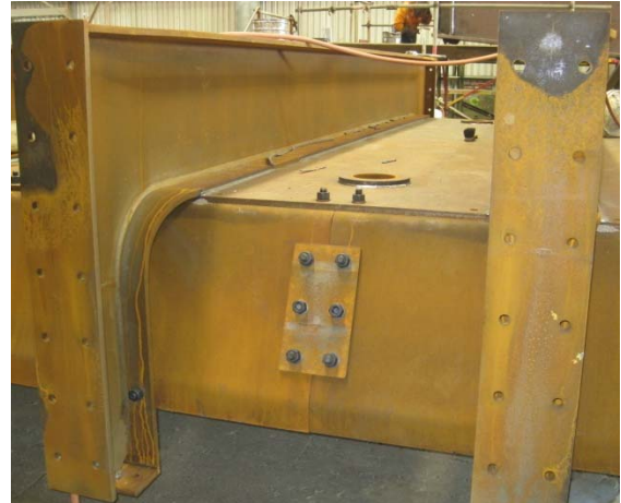
Figure 7: Inverted view of the cross beams welded to the deck during fabrication. The kerb plates are bolted to the deck plate and to the cross beam up stands.
