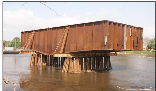
**Figure 4:** Storage of Haunched Steel Girder Pier Segments on Custom Built Racks in River
