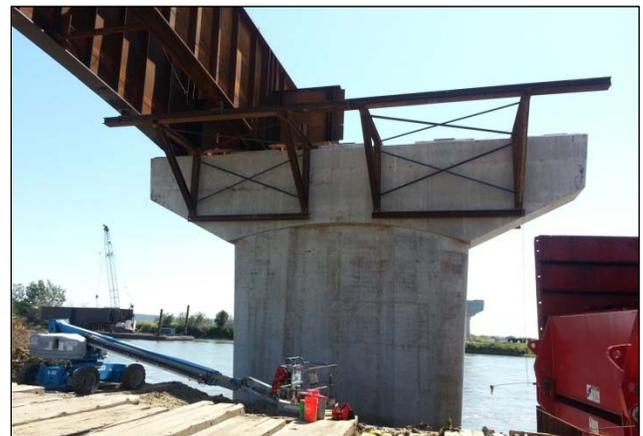
**Figure 6:** Temporary “Wing” Struts for Interior Pier Steel Section Support During Erection
