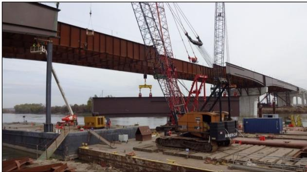
**Figure 7:** Erection of Drop-In Steel Segments at Main Span
