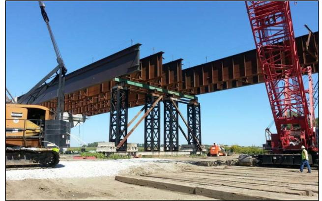
**Figure 5:** Temporary Bents Utilized During Girder Erection of the Main Steel Unit
