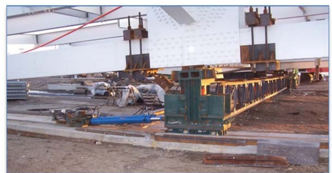
Figure 3 Launching System
