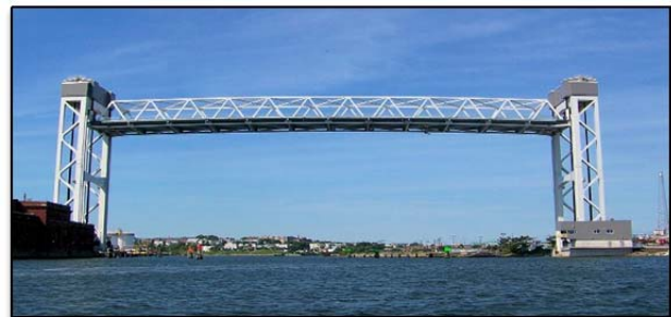
Figure 2 Chelsea Street Bridge Replacement
