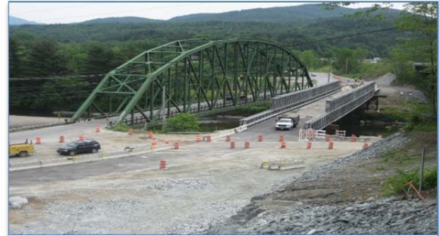
Figure 8 Checkered House Bridge Prior To Renovation
