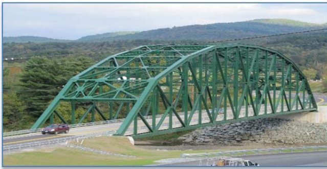
Figure 9 Bridge After Renovation
