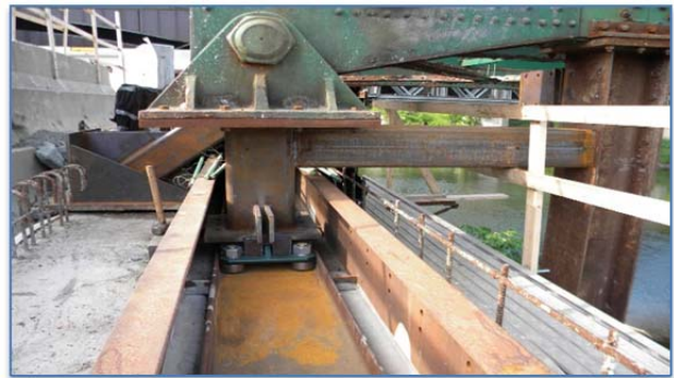
Figure 10 Launching System
