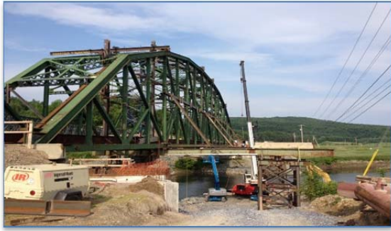
Figure 8 Falsework
