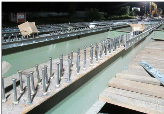
Figure 1. Steel girder with closely spaced studs
