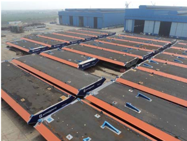
Figure 5 – Fabricated box girders ready for load-out.
