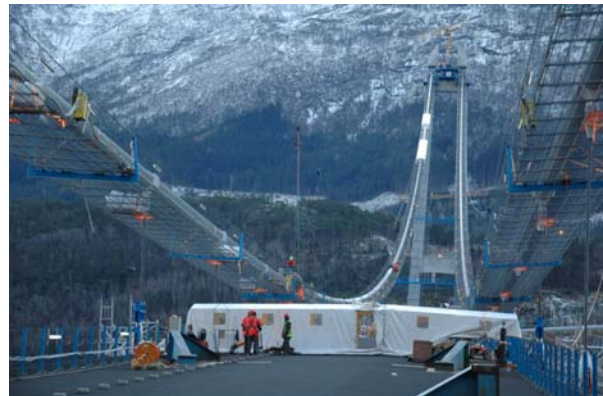
Figure 7 – Welding of box girder joint inside tent.
