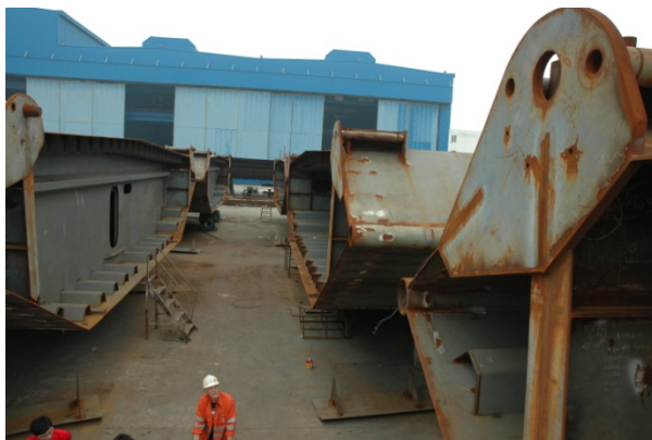
Figure 9 – Box girder sections at fabrication yard with assembly brackets at the upper deck edge.
