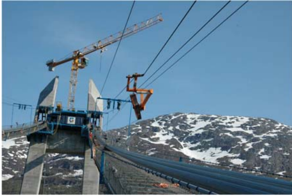
Figure 4 – Spinning wheel travelling from the pylon with 4 loops of wire.
