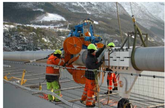
Figure 10 – Cable wrapping in process.
