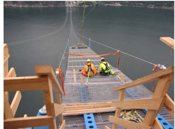
Figure 3 – Catwalk netting under construction
