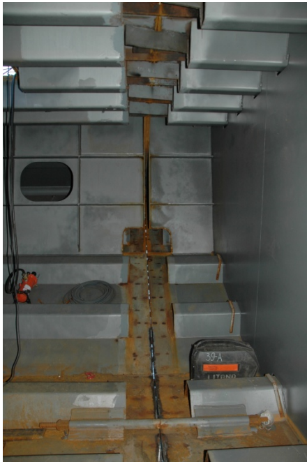
Figure 8 – Box joint at start of welding process
