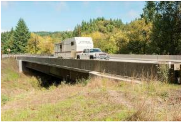
Figure 9 - Dodge Creek Bridge in service.
