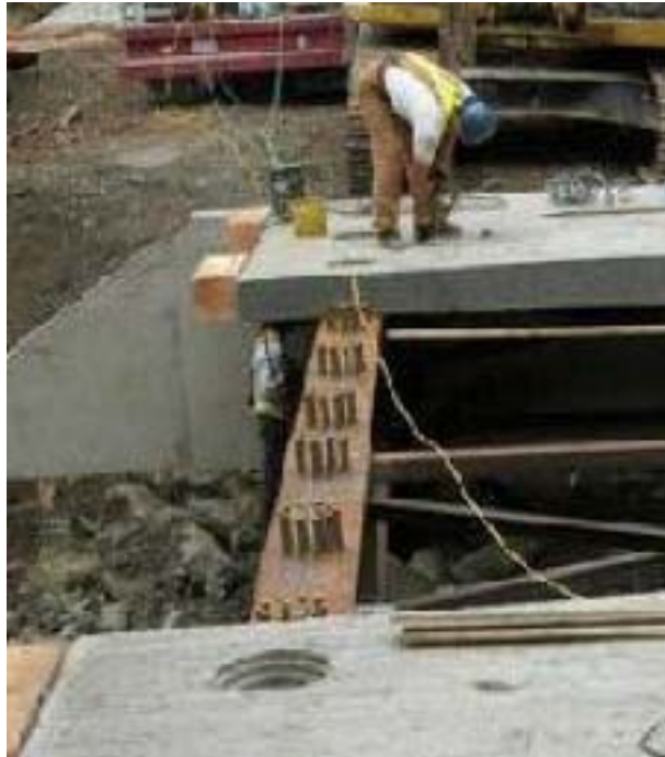
Figure 1: Shear stud clusters [7].
