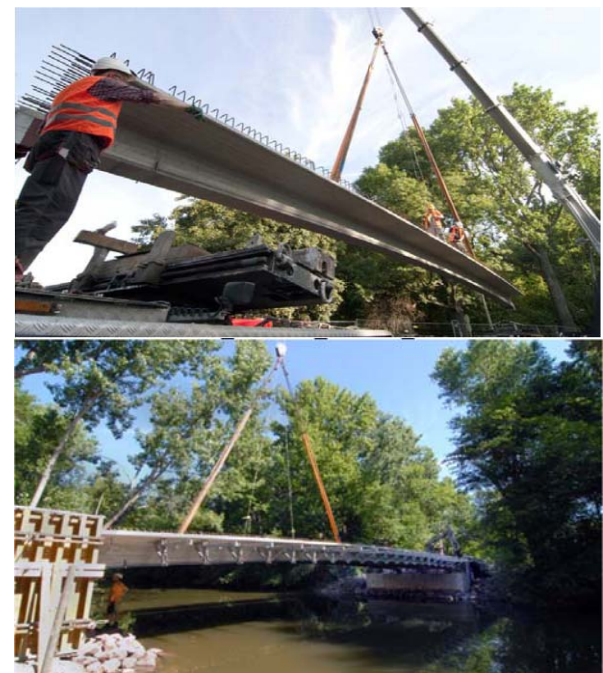
Figure 27: Erection phases BW 49
