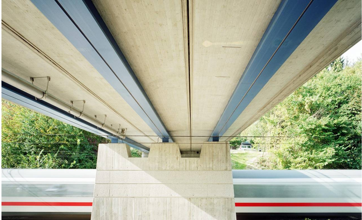
Figure 1: View beneath Pöcking Bridge (Germany) with Precobeam elements
