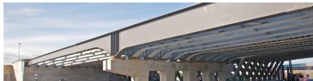
Figure 2: Metallized interchange rehabilitation project in Québec City (courtesy of Canam-Bridges)
