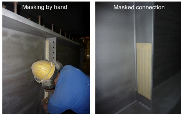
Figure 1: Masking of connection faying surfaces (courtesy of Canam-Bridges, Québec)
