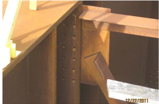
*Figure 22. Typical Cross Frame Connection (shown prior to bolt installation).*
