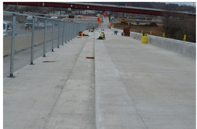
Figure 18. Longitudinal Deck Closure Pour (note construction joints).
