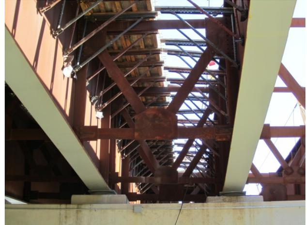
Figure 17. Typical Cross Frame in Closure Bay.
