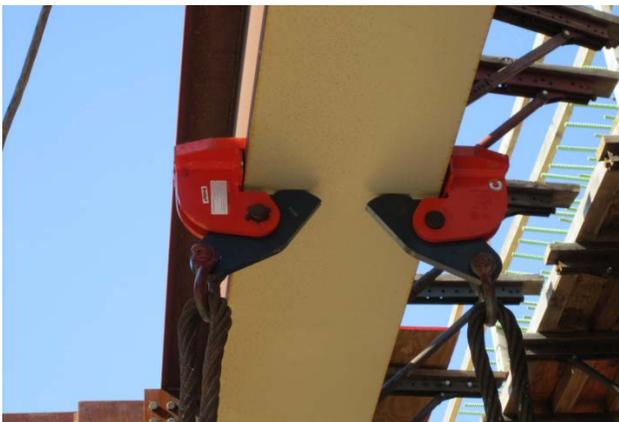
Figure 14. Beam Clamp Supporting Block Weight.
