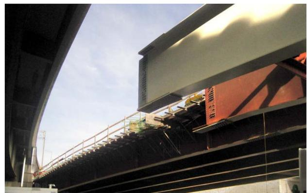
Figure 6: Cantilevered Ends of G1 and G2.
