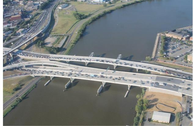
*Figure 2. New 11<sup>th</sup> Street Bridge Separates Local from Interstate Traffic.*
