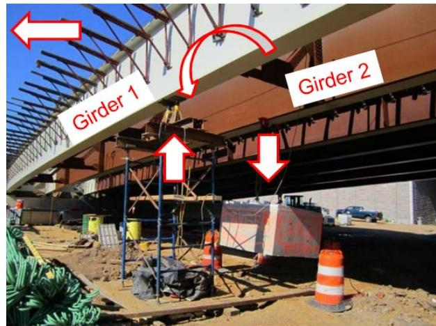
Figure 15. Jack and Block Weight Counteracting Two-Girder System from Rotating (arrows showing outside of curve, direction of girder rotation, and counteracting couple from temporary loads).
