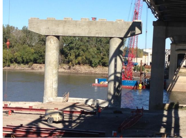
Figure 9. River Bent Construction
