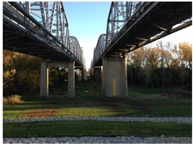
Figure 2: Existing Platte Purchase Bridge (left) and Fairfax Bridge (right)
