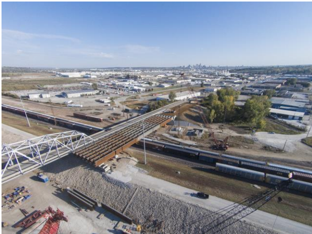
Figure 8. Steel Erection over the Railroad Tracks
