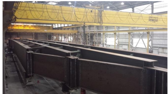
Figure 11: Photo from Shop Assembly
