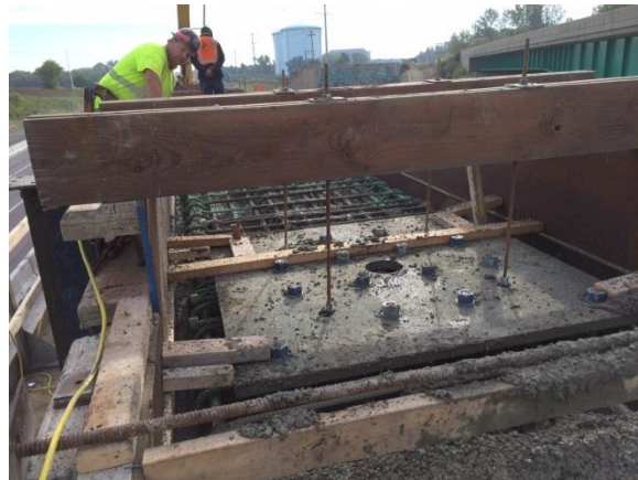
Figure 17: Table Top Bearing Plate
