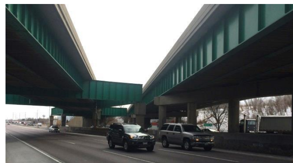
Figure 1: Existing Higgins Road Bridges
