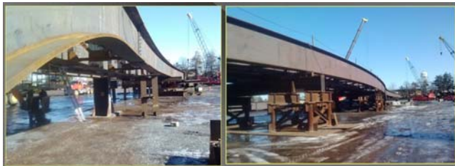
Figure 11 – Intermediate Falseworks
