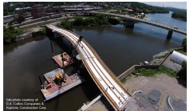
Figure 19 Forming the Deck
