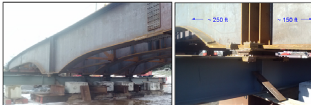
Figure 10 – Temporary Fixed Pier, Bearing
