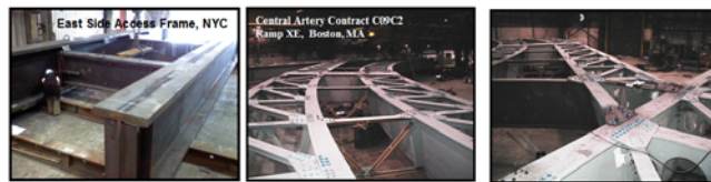
Figure 15 – Indoor/Pre-loaded Assembly (usually only feasible for smaller-footprint bridge structures)
